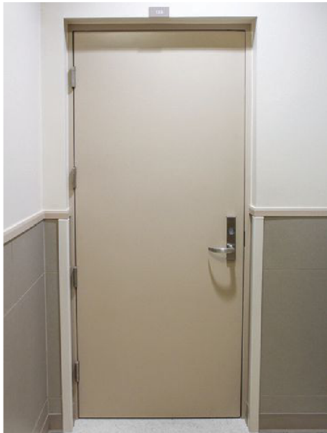
Tornado safe room doors need to be tested and certified based on the specific assembly of the door panel, the door frame, and the hardware used, even when used in rooms that double for other uses.
