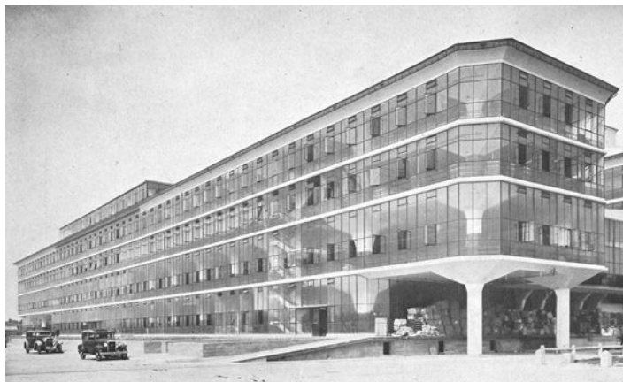
The Van Nelle Factory in Rotterdam by Brinkman and Van der Vlugt (1930) was published in RECORD in 1929 and 1931 (opposite, top). It is known for the sweeping arc of its expansive glass curtain wall facade. Inside, poured-in-place concrete mushroom columns support floor slabs (opposite, bottom). The Boots factory in Beeston, England, by engineer Sir E. Owen Williams (1932; in RECORD 1933) was designed to expand when needed (above). It too has a concrete mushroom column frame and glass curtain walls (left).
