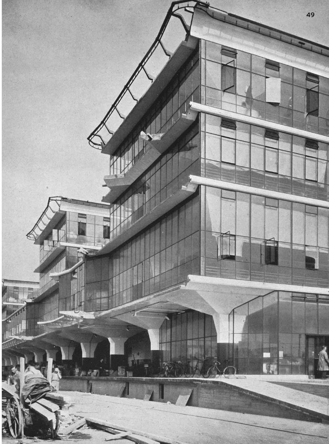
The Van Nelle Factory in Rotterdam by Brinkman and Van der Vlugt (1930) was published in RECORD in 1929 and 1931 (opposite, top). It is known for the sweeping arc of its expansive glass curtain wall facade. Inside, poured-in-place concrete mushroom columns support floor slabs (opposite, bottom). The Boots factory in Beeston, England, by engineer Sir E. Owen Williams (1932; in RECORD 1933) was designed to expand when needed (above). It too has a concrete mushroom column frame and glass curtain walls (left).
