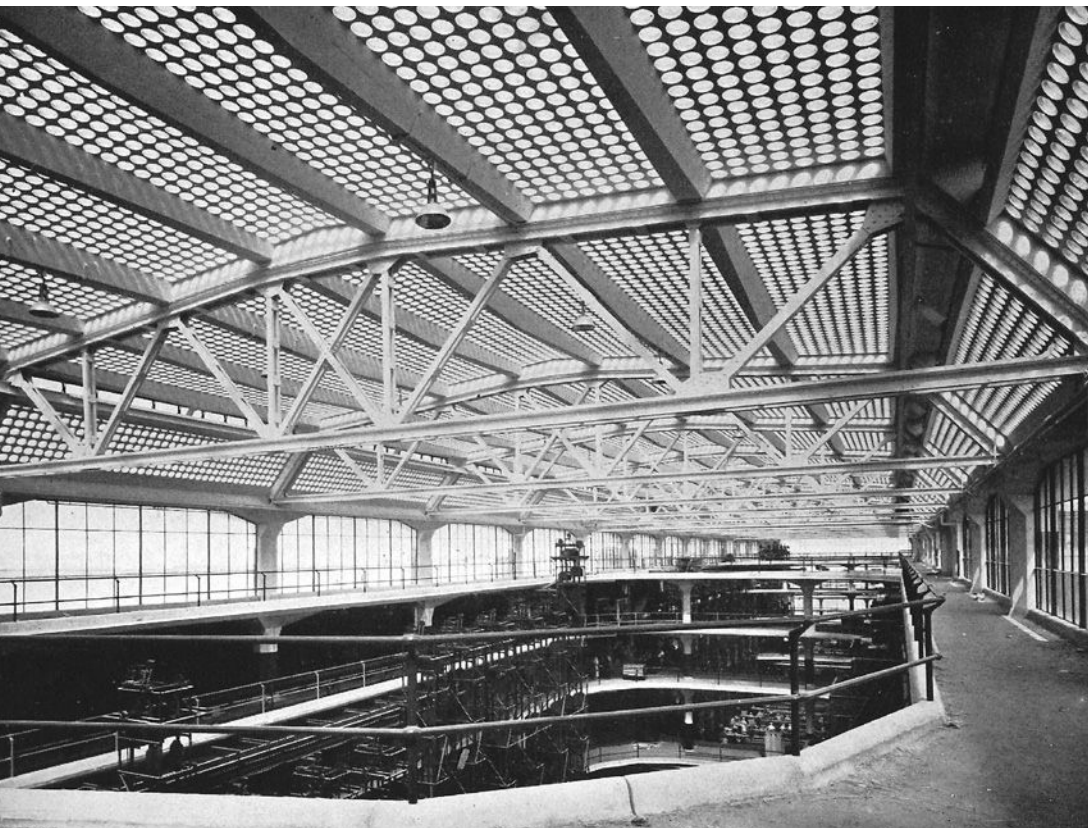
The interior of the Boots factory (RECORD 1933) features a dramatic translucent roof (left) with circular glass discs embedded in wire-reinforced concrete. The general offices of the Van Nelle Factory (left, below) contained glazed conversation booths that allowed daylight to penetrate while still affording privacy to the employees; today the factory is an incubator for arts organizations.
