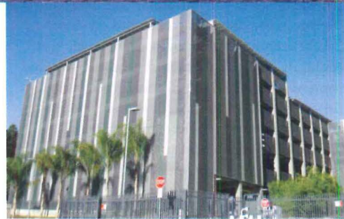
The textile facade on the new FBI offices and parking garage in San Diego provides an intriguing and elegant appearance that blends in well with the surroundings while meeting the client needs for security.
