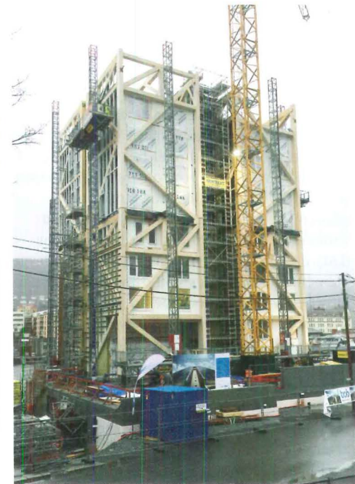
NORWEGIAN WOOD The Treet tower (left and below) in Bergen, Norway, is slated to be the tallest timber building when completed later this year. It consists of prefabricated CLT apartment units stacked within a structural frame of glulam trusses. The units sit on “power stories”—levels reinforced with precast concrete slabs that occur every fifth floor.
