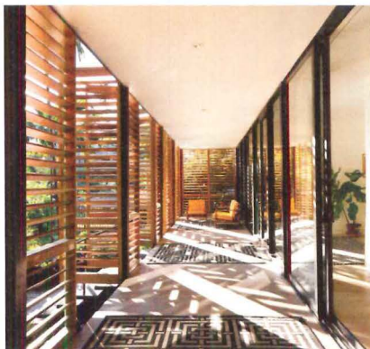
Red cedar folding shutters extend across the house's front facade (top). The screen masks a 50-foot-long porch (above, left) that repeats along the rear. Inside, the open-plan interior (above, right) has expansive views of the jungle-like setting.
