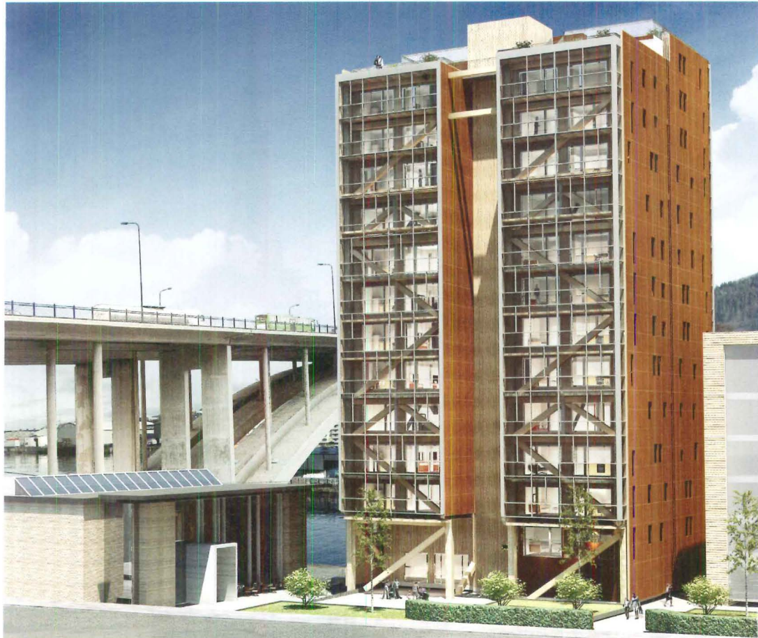
NORWEGIAN WOOD The Treet tower (left and below) in Bergen, Norway, is slated to be the tallest timber building when completed later this year. It consists of prefabricated CLT apartment units stacked within a structural frame of glulam trusses. The units sit on “power stories”—levels reinforced with precast concrete slabs that occur every fifth floor.
