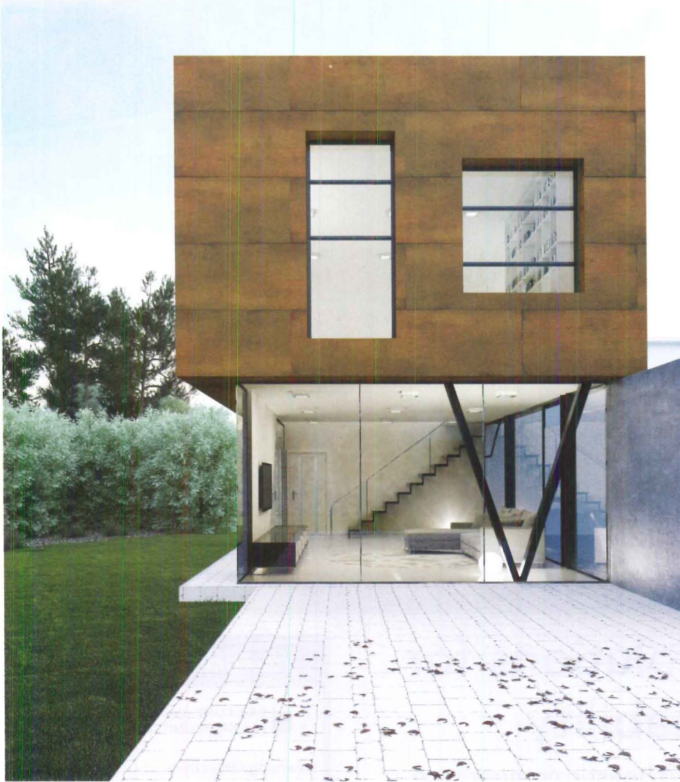
Ceramic tile—used on this house with a simulated steel finish—has been analyzed by Tile of Spain with an industry-wide, generic LCA to show its low long-term environmental impact.
