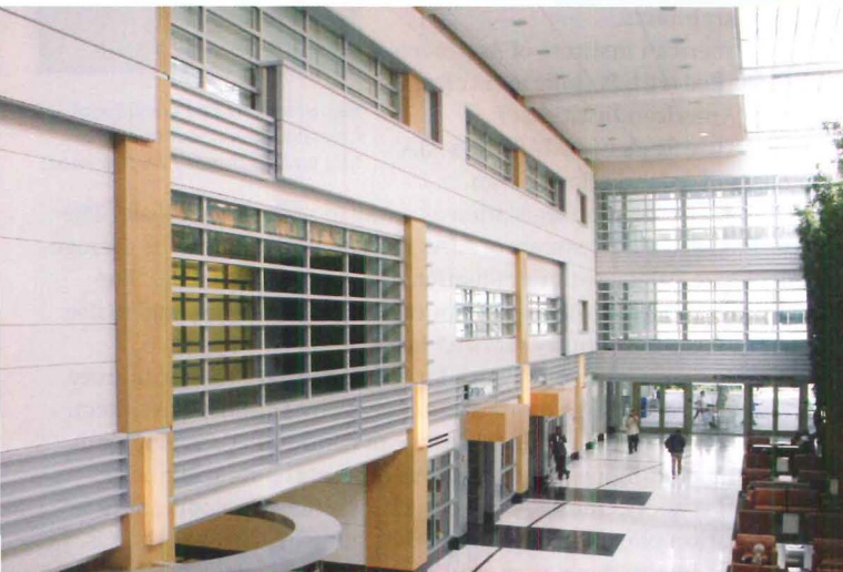
Stantec UC Davis Medical Center in Sacramento, CA Interior Walls
