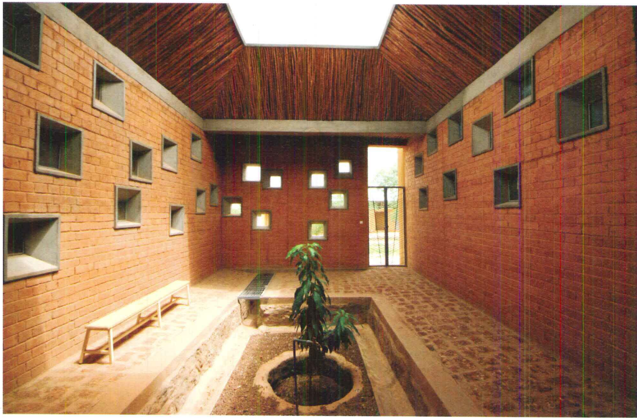
Locally produced clay bricks form the inner walls of the building (this page). Square, operable windows aid in natural ventilation and frame views of the landscape for patients (this page and opposite).
