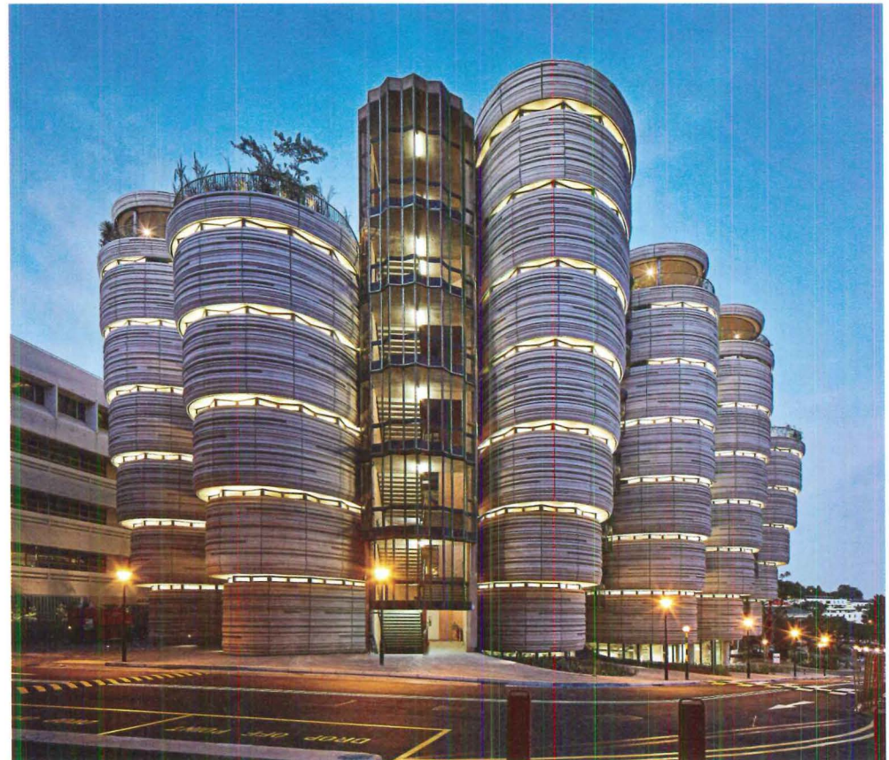
The Learning Hub for Nanyang Technological University in Singapore opened early in 2015. Heatherwick worked with local architects, CPG Consultants, on the design for the poured-concrete cluster of eight-story zucchini-shaped towers.
