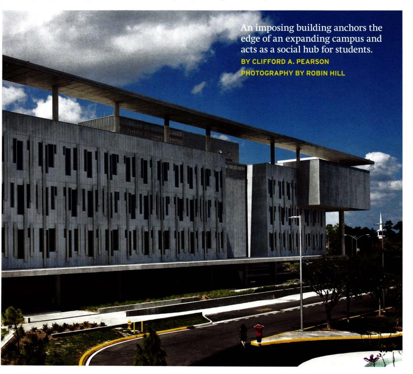
SUN BLOCK On the south elevation, the architects used precast-concrete panels with two different textures to provide subtle contrasts to the poured-concrete frame. Vertical strips of metal help shade narrow windows from the sun, while a long concrete canopy on columns protects a roof terrace where the college can host parties and special events.
