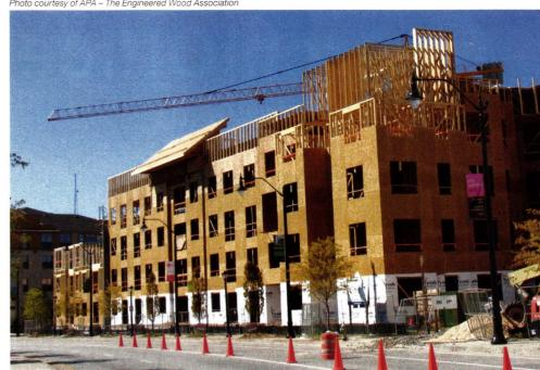
The exterior, sealed sheathing air barrier approach meets the key requirements of an effective air barrier system—i.e., that all elements (materials) be air-impermeable, that it be continuous throughout the building enclosure, structurally adequate and sufficiently rigid, and that it have a service life as long as that of the wall and roof assembly components.
