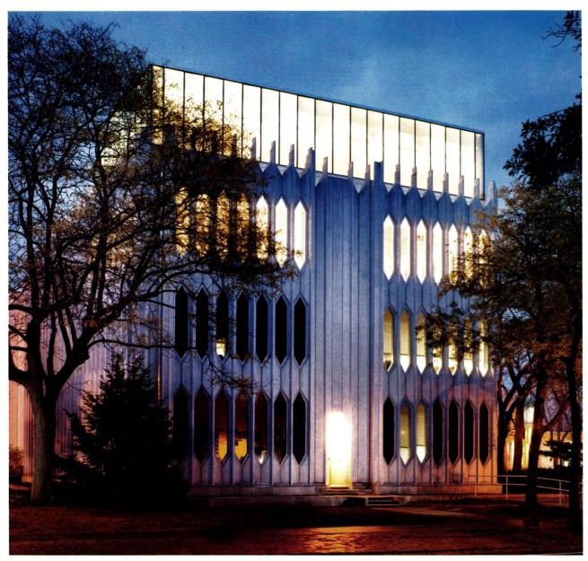
ALL AGLOW Cutting open a section of the roof at one end of Minoru Yamasaki's three-story Bibbins Hall allowed Westlake Reed Leskosky to insert a glass-topped volume for musical performances within the building's original load-bearing precast-panel shell (opposite). After dark, the room's new clerestory functions as a lantern (left).
