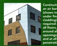
Continuity of an air barrier (shown in blue under final cladding) is required across all floors, around all openings, and at all penetrations.
