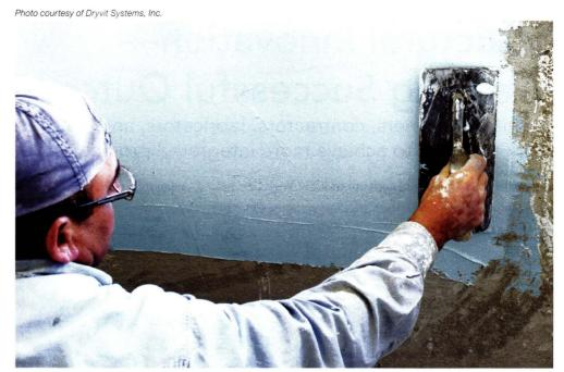
Fluid-applied membrane systems can be applied to an appropriate substrate by using a trowel, a roller, or a sprayer as field conditions may warrant.
