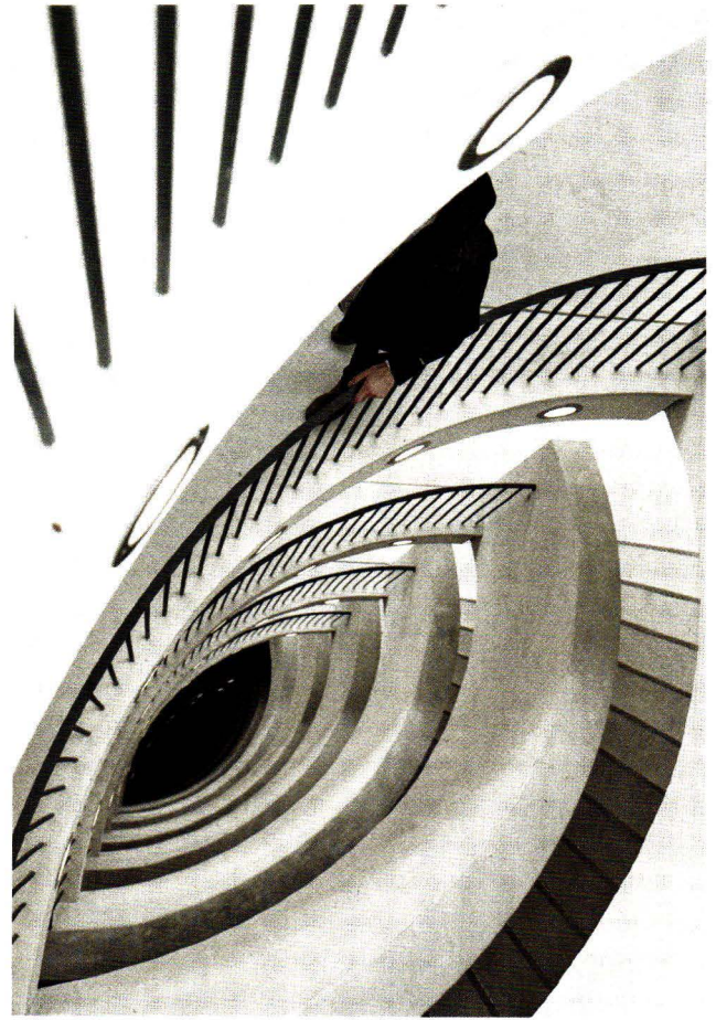
GEOMETRY LESSON The precisely aligned bamboo stalks are spaced 9 inches apart and affixed to the precast-concrete structure with custom curved metal brackets on steel bars (left). The striking eye-shaped poured-in-place concrete staircase invites users to ascend and descend the various levels on foot (above).
