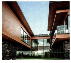
Aldea Homes designed and constructed this house in Burnaby, BC, Canada, using Longboard aluminum soffit and siding in place of wood.
