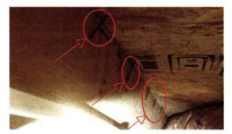
Fasteners missing joists create squeaky floors and expensive callbacks. A fastening guide helps installers.
