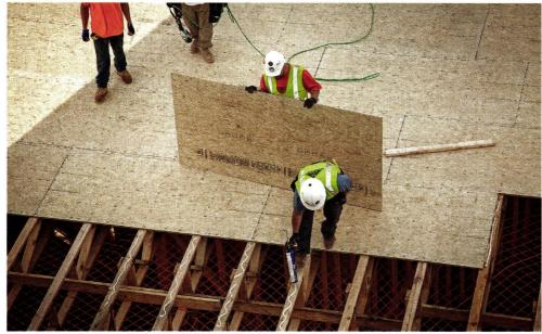
Both glue and mechanical fasteners should be used for a solid installation.
