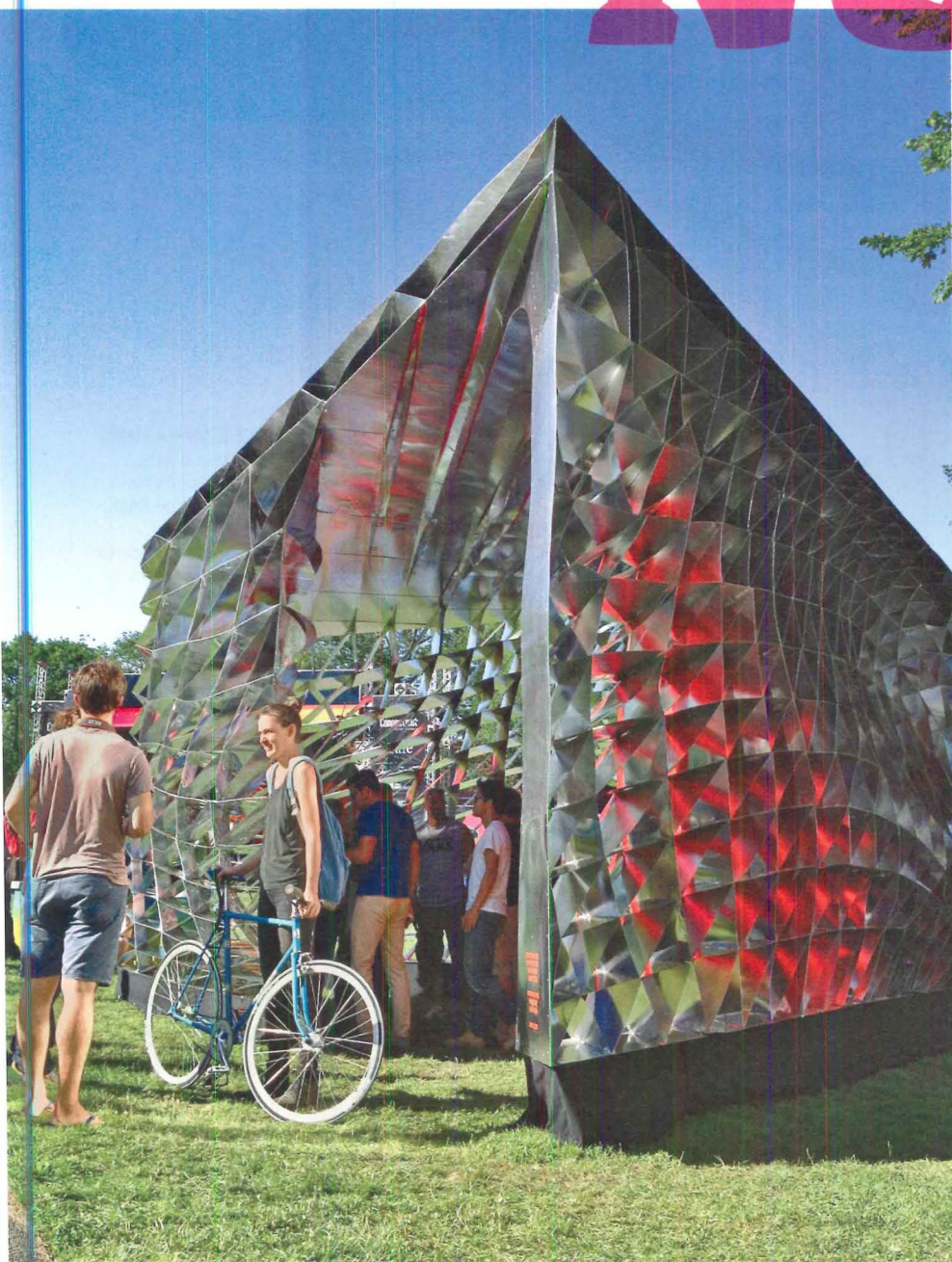
FULL METAL JACKET The School of Architecture students at Yale University designed and built a colorful aluminum-paneled information center for an arts festival in New Haven in 2012.
