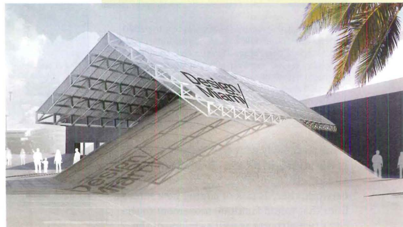
The 500-ton pile of sand that forms part of the pavilion, dubbed Tent Pile, will be 70 feet wide at its base.
