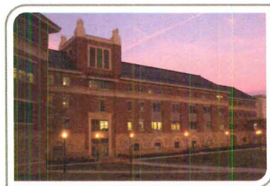
before 150W High Pressure Sodium Lamps
