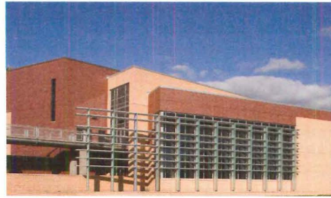
Fixed exterior shading devices like the ones shown here cannot adjust to changing weather and light conditions.
