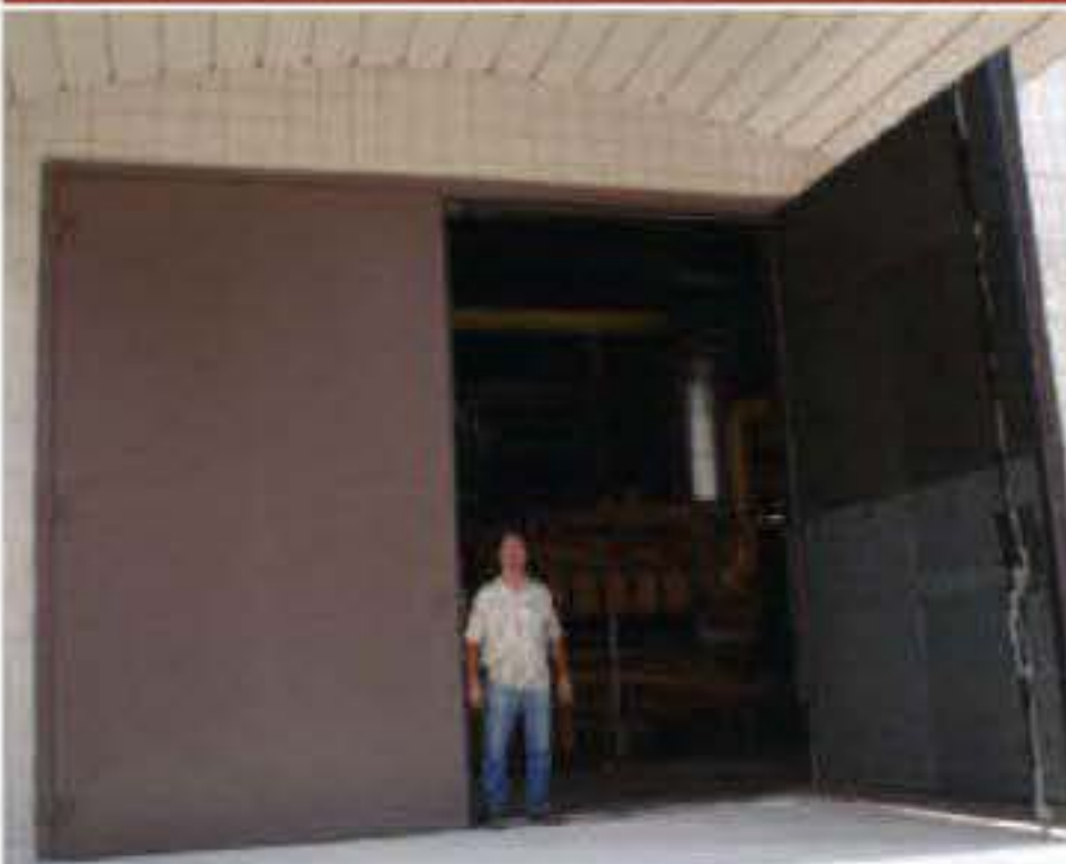
Oversized door 188 in. by 158 in. with STC 55 rating.
