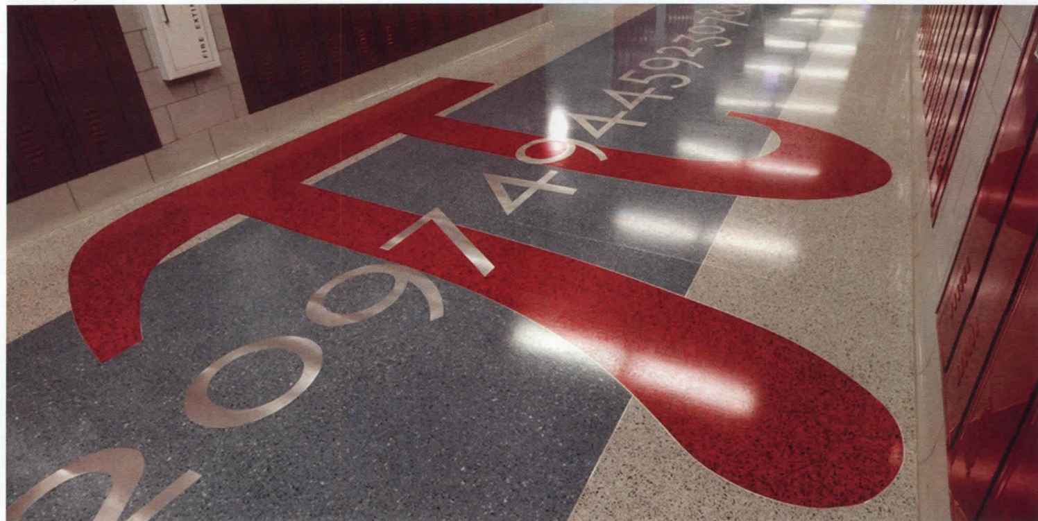
Corridors in Chicago’s West Ridge Elementary School are cast in terrazzo with ornamental motifs. Metal divider strips are used to separate different terrazzo colors to produce the floor designs.
