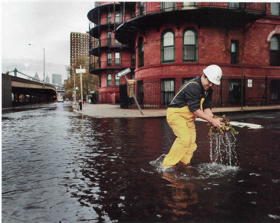
A New York City worker clears a sewer drain in Lower Manhattan after Superstorm Sandy.
