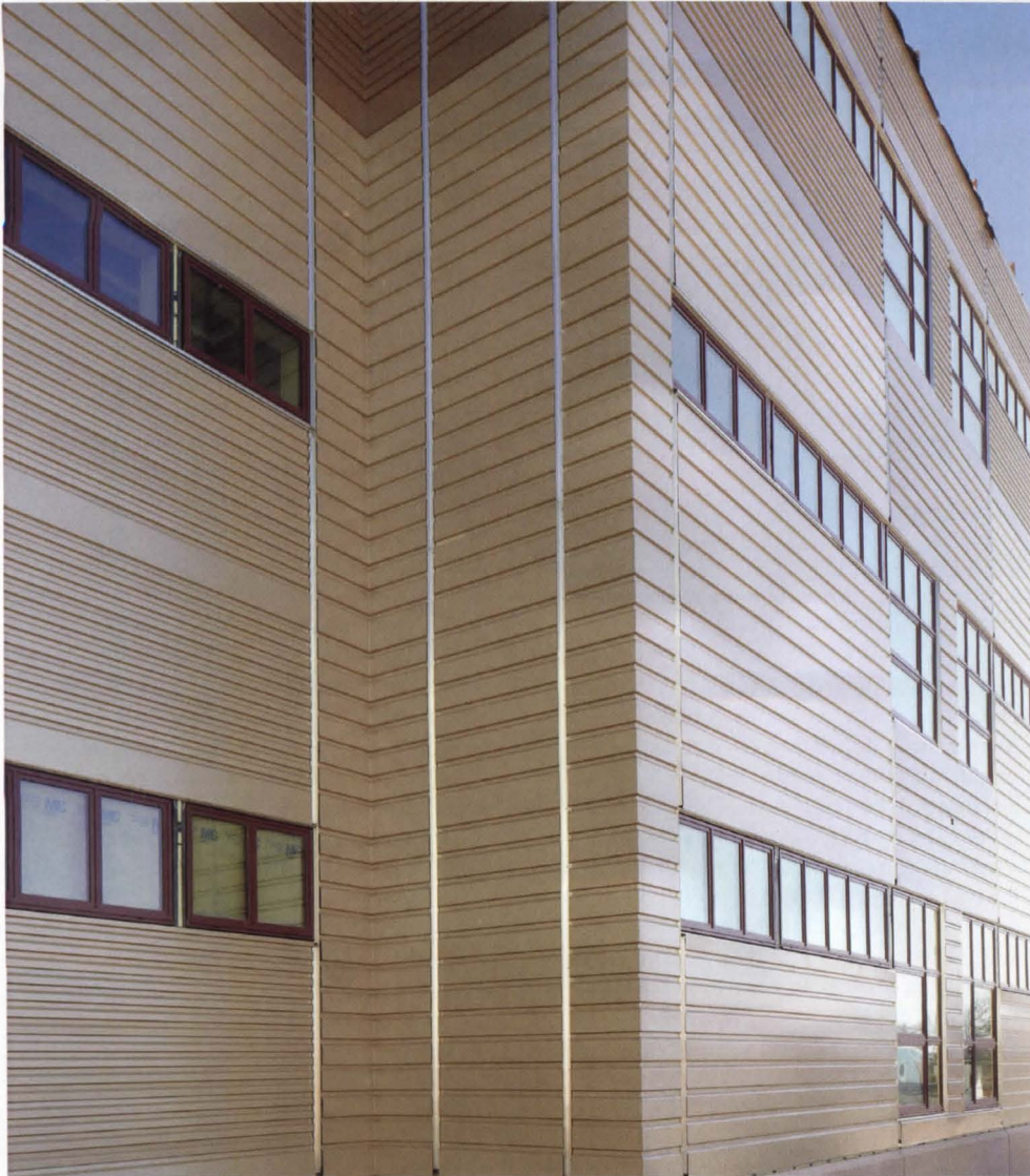
This middle school received a 3-inch insulated panel system, which provides an R-value of 21 on top of the insulating value of the wall beneath, which helps schools endure harsh winters and save energy without requiring excessive façade maintenance.
