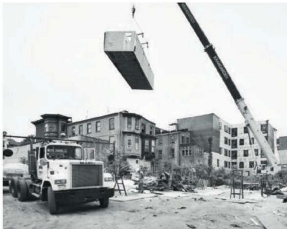
BUILDING BLOCKS The Modules' prefab units took just over four weeks to install (left). The project stands across from a low-rise public housing project and is flanked by brick buildings (below). Signage on the project's west elevation (right) advertises its modular components.
