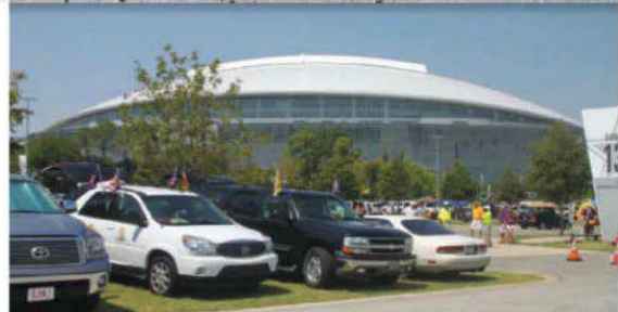
PaveGro was installed at the Cowboy Stadium as an aesthetic and environmentally friendly answer to overflow parking.
