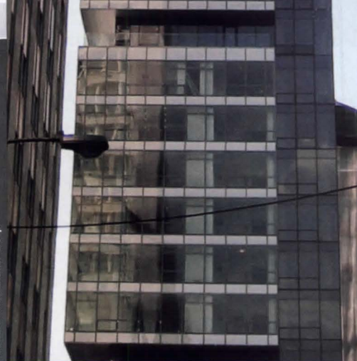
Trump Taj Mahal New Hotel Tower, New Jersey Architect: Friedmutter Group
