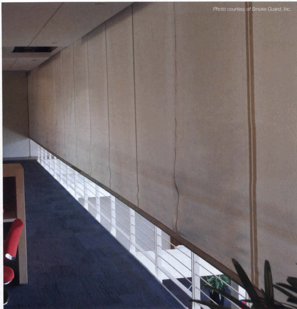
This example of a large-opening automatic flexible smoke-rated curtain has zero percent residual opening when activated and employs a gravity fail-safe system.
