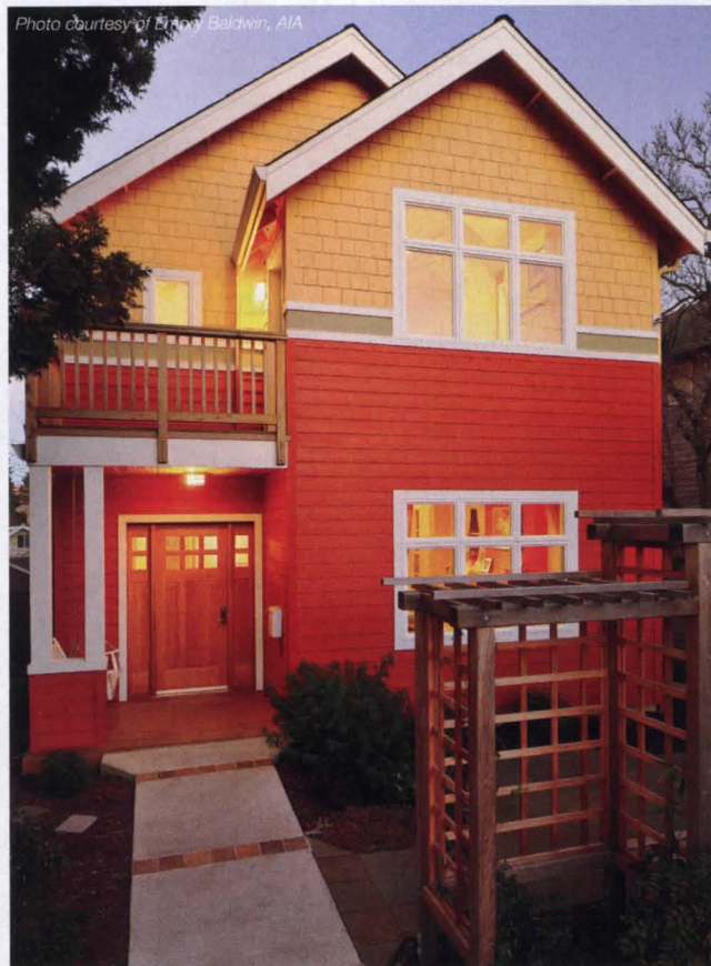
Photo courtesy of Gunnar Baldwin, AIA Universal Design solutions can be "invisible" and an accessible house can be a multi-story structure on an urban lot.
