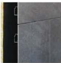
Porcelain cladding installed with Marazzi's Ventilated Wall System
