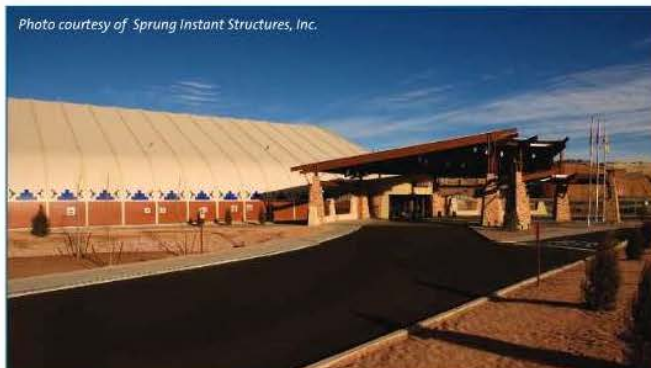
Photo courtesy of Sprung Instant Structures, Inc.
