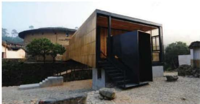
The Bridge School, by Li Xiaodong Atelier, is located in a remote village in China.
