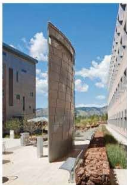
The RSF's bid for LEED Platinum includes site strategies such as permeable pavement in courtyards and gabion walls made from rock recovered during excavation for the foundations.
