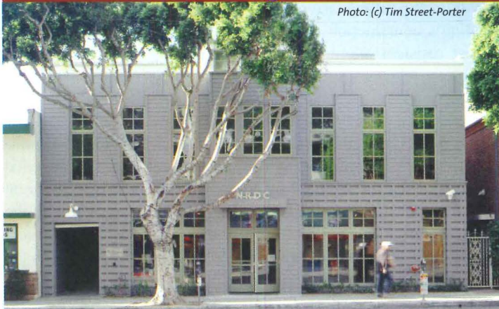
The Natural Resources Defense Council — Robert Redford Building is clad in durable fiber cement siding, that contributed to its LEED® Platinum rating.
