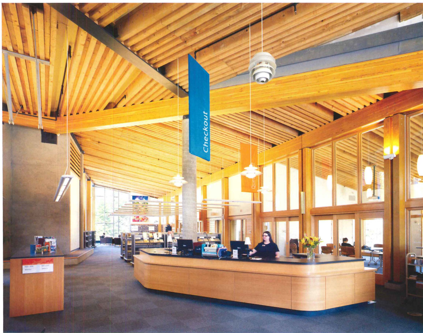
The architects developed a system of laminated-wood construction for a ceiling of repetitive bands of rich mahogany-hued hemlock, robust enough to support the green roof and the snow. The main area of the library accommodates the entry sequence, the circulation desk, and the stacks.
