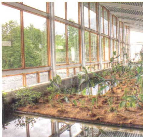
The Omega building houses aerated lagoons where the roots of wetland plants act as habitat for microbial populations that scrub the water.
