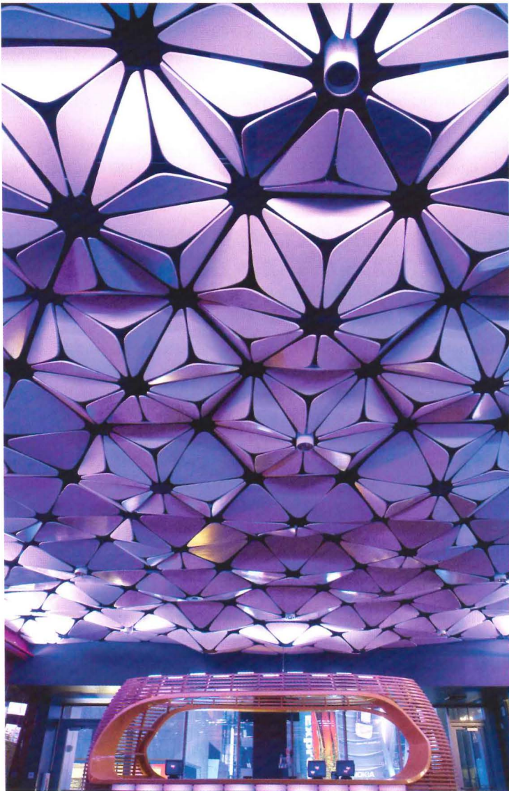
The ceiling's bold design lures visitors up a stairwell to the second-floor club (above). Light fixtures and sprinkler heads are hidden within the center of the ceiling's flower shapes (left). The straps used to tie each flower to the next must withstand a certain tolerance of rotation (below).
