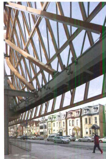
The two ends of the new Dundas Street facade (opposite) offer places to hang banners. This curving glass, steel, and wood elevation addresses the scale of houses across the street (below). A “barnacle” stair cantilevers off the facade overlooking Grange Park (left).
