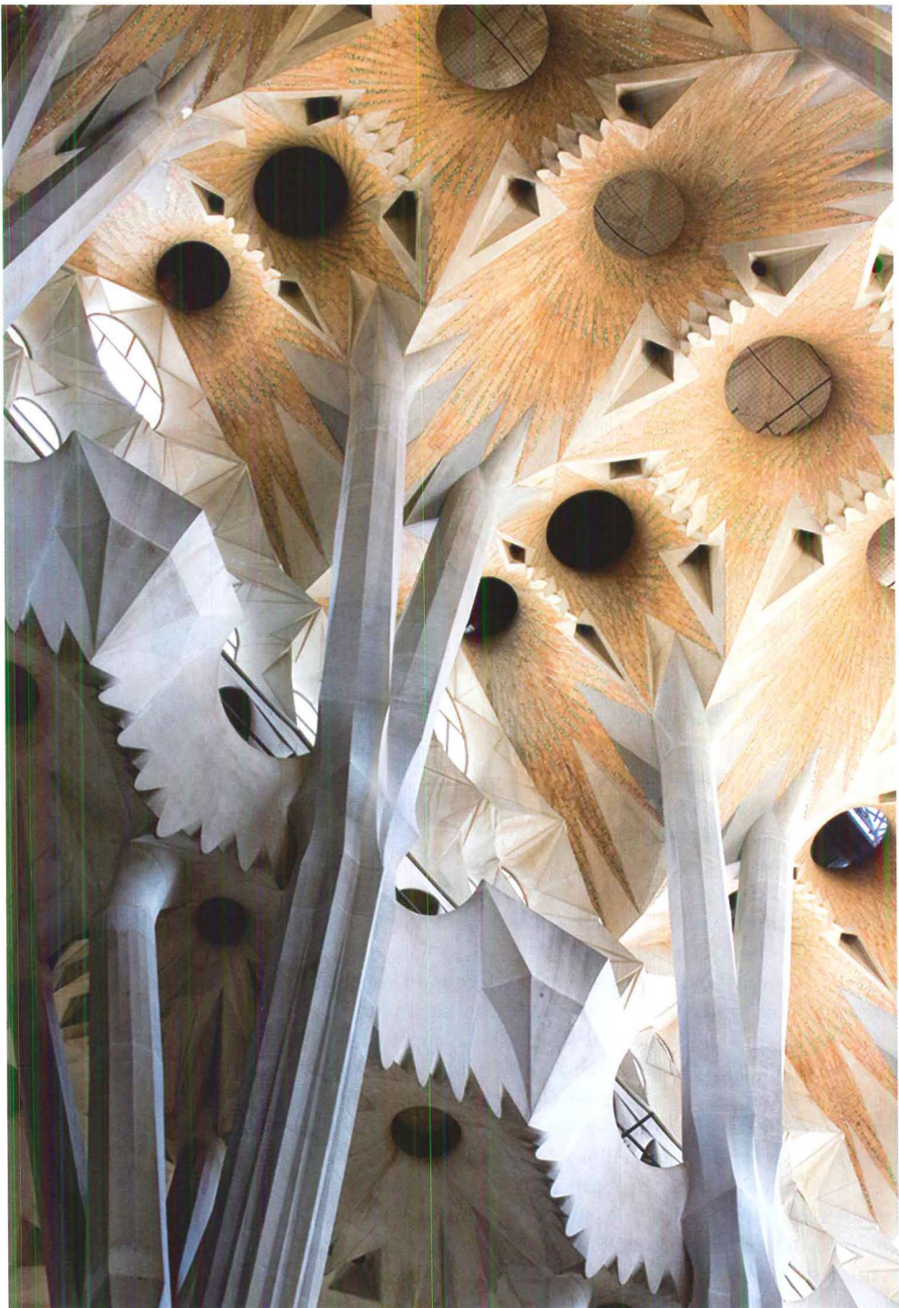
Lluís Bonet, one of the architects charged with reconstructing Gaudí's models after they were burned during the Spanish Civil War, shows his vision for the church (below). The hyperboloids of the nave ceiling use traditional Catalan vaulting techniques (right).
