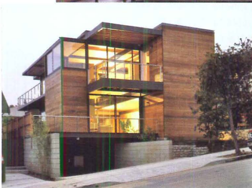
Designed for LivingHomes founder Steve Glenn, this house was built over eight hours on April 13th, 2006, from 11 prefabricated modules – each weighing an average of 10,000 pounds.
