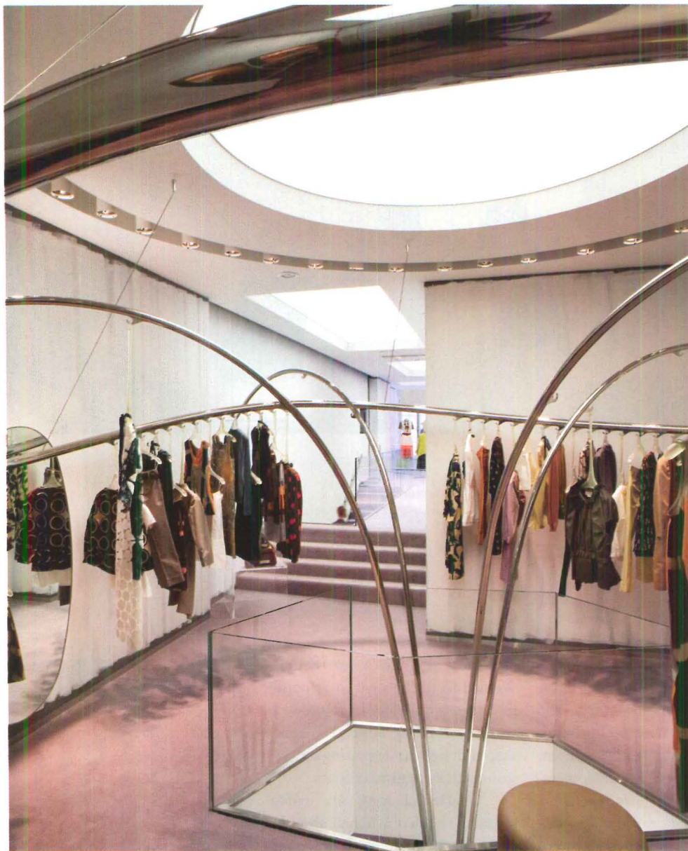
Track-mounted PAR30 halogen lamps are installed around a circular fluorescent luminaire and adjacent to the stair to highlight individual items (left and bottom). Large, round luminaires with opalescent glass diffusers illuminate the first-floor galleries (above).
