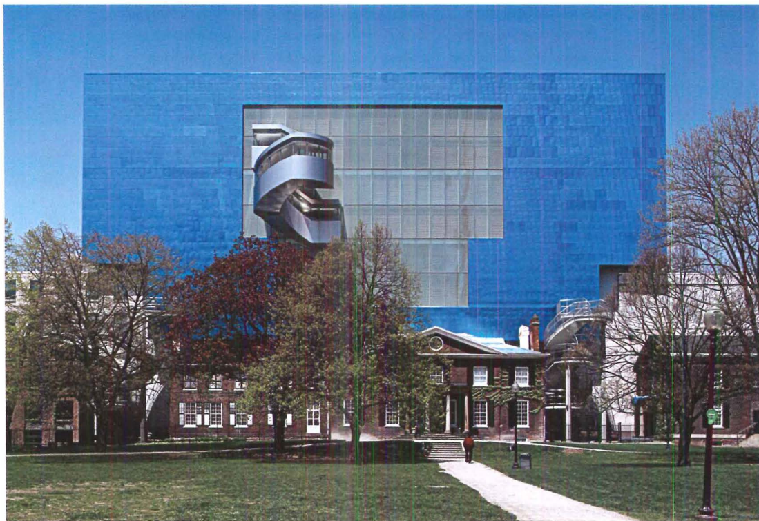
The two ends of the new Dundas Street facade (opposite) offer places to hang banners. This curving glass, steel, and wood elevation addresses the scale of houses across the street (below). A “barnacle” stair cantilevers off the facade overlooking Grange Park (left).
