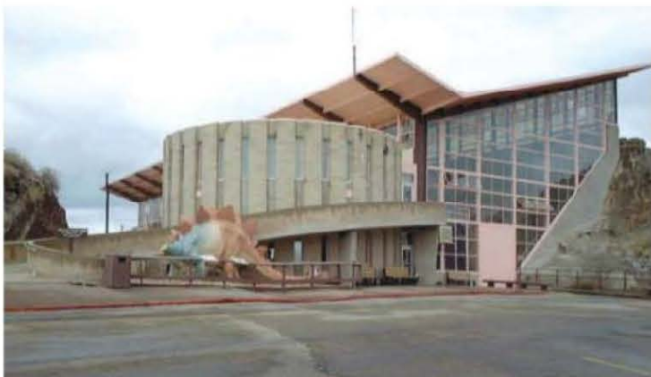
Part of the Quarry Visitor Center, by Anshen and Allen, will be torn down.
