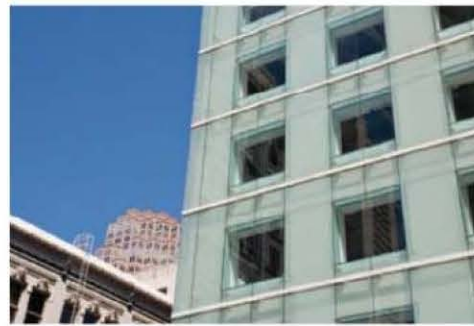
Glass frames span the 9-inch gap between the fritted-glass wall and the original brick facade. Clear glass is used over the existing window openings (above and right).
