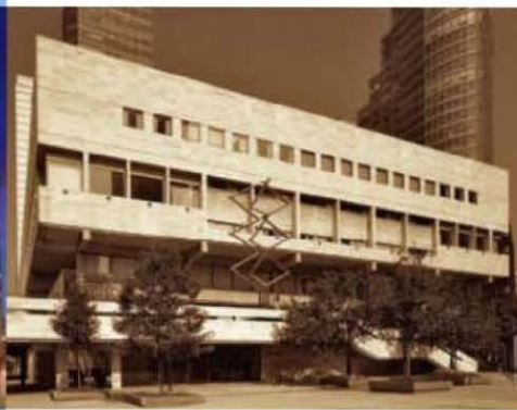
The new expansion and renovation of Pietro Belluschi's 1969 original (left) involved adding a wedge-shaped addition (opposite) with new travertine on West 65th Street, and glazing (far left) on Broadway.
