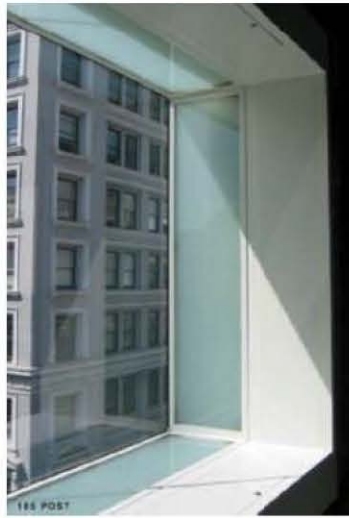
Glass frames span the 9-inch gap between the fritted-glass wall and the original brick facade. Clear glass is used over the existing window openings (above and right).
