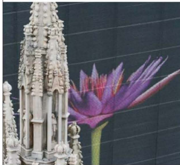
Mediamesh® at the Piazza Duomo, Milan, with programmable, embedded LEDs.
