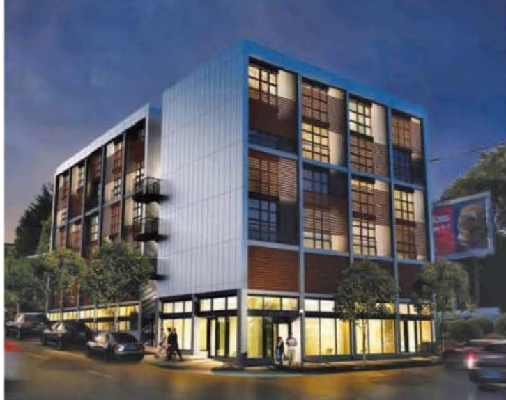
151 Lofts, Seattle, 2010 The design for this 18-loft-unit building includes 5,600 square feet of commercial space and features solar shading, green roofs, and natural ventilation.
