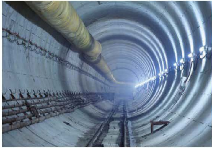
Rebuilding the nation's sewers should be part of the stimulus program.
