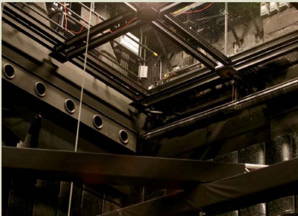
The wire grid ceiling over the studios provides a walkable surface and structure from which to hang banners, diffusers, and 360-degree screens for immersive performances (left). Computer-milled acoustical panels in the studios have random, pocked surfaces (above) and are lined up along the studio walls (below left). Live sound testing is performed on a mock-up of the panels (below).
