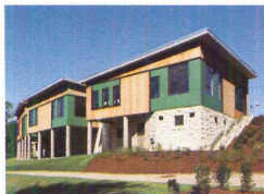
56 Hazelwood School, Glasgow, Scotland GORDON MURRAY + ALAN DUNLOP ARCHITECTS
