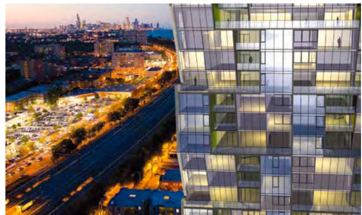
At Solstice on the Park, low-E glass is angled to reduce its reflective quality.
