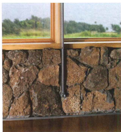
Steel supports (left) tie the structure down to the lava-rock base. Custom details include rolling doors (below left) that open the walls to wide Pacific views, as in the kitchen/dining area (above).
