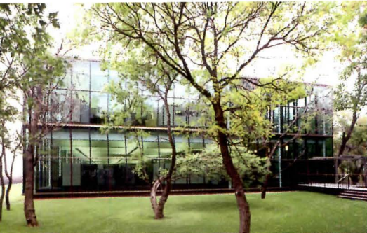
Julie Snow Architects Great Plains Software Development Building, Fargo, N.Dak., 2001
