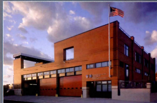
Karahan & Associates Combined Fire and Emergency Medical Service Station, Rockaway, N.Y., 2004
