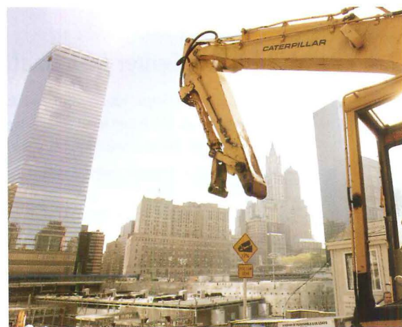
Freedom Tower construction under way in April.
