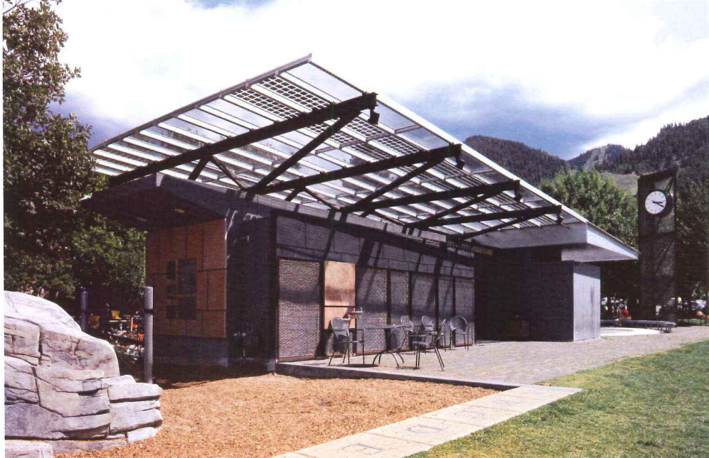
Aspen’s Wagner Park Edge includes a glass-laminated photovoltaic installation as its sole power source (above and right).
