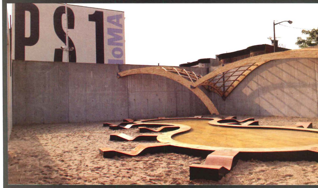
OBRA Architects' courtyard canopies, constructed of plywood and polypropylene, shelter hundreds of visitors to P.S.1's Saturday parties, when the crowds are avoiding the sun (above) or wading through one of the wood pools (below).
