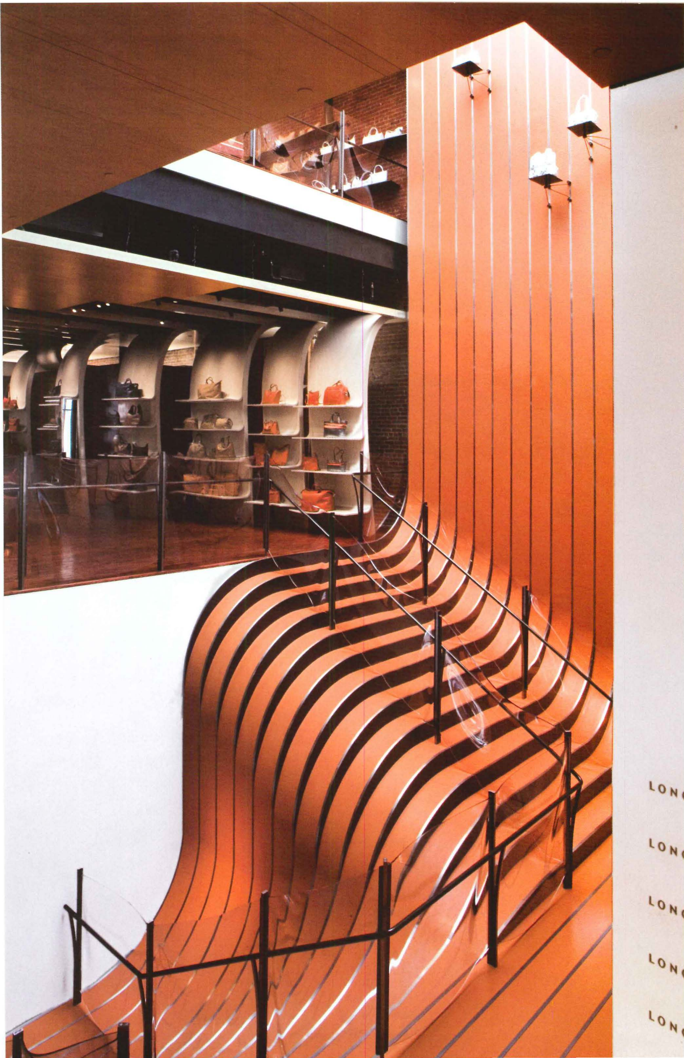
For the new stair (left and opposite two), Heatherwick Studio carved a 46-by-27-foot atrium, rising 60 feet, into the existing building. A skylight helps draw people upstairs. The designers used a thermoplastic material, instead of glass, to create the sensuously curving balustrades. Each of the 57 panels is unique.
