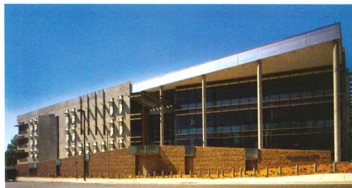
The U.S. Federal Building was constructed after the Oklahoma City bombing.
