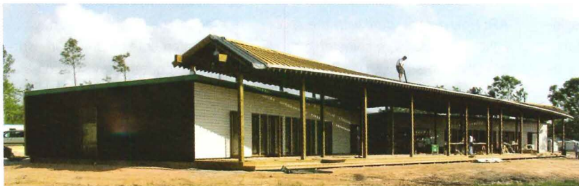
A crew completes work on two SHoP-designed buildings unified by a sculptural canopy.
