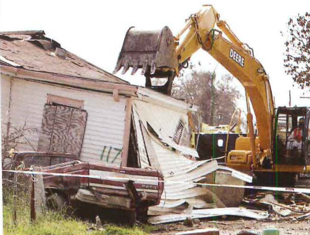
Demolition in the Lower Ninth Ward.
