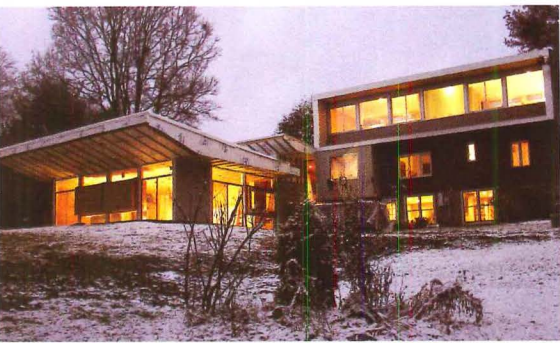
Wyoming Loft Addition, Cincinnati, 2006 Renovation to a Cincinnati-suburban bungalow comprising a bedroom and bath connected to the main floor by a new light-well and stair. A ground-floor addition contains living, dining, kitchen, and support spaces.
