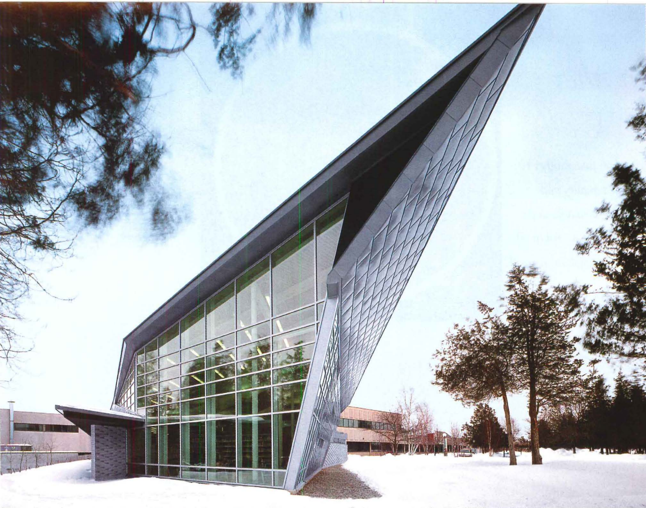
Loyalist College, Belleville, Ontario, Canada; Architect: Stephen Teeple Architects, Toronto, Ontario, Canada; Flat Lock Interlocking Wall Tiles; Fabrication and Installation: Simple Gooder, Toronto, Ontario, Canada
