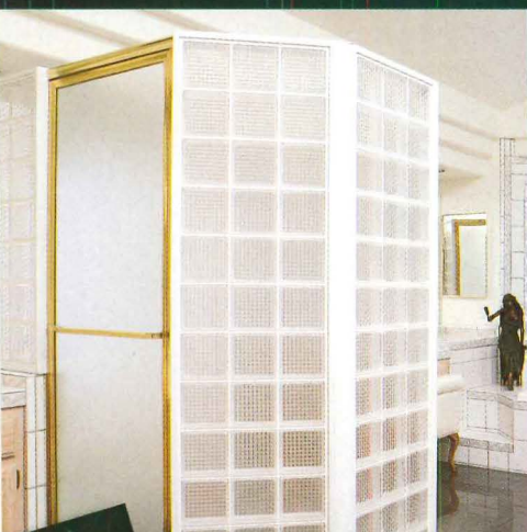
45-degree corner caps were used to connect Hy-Lite acrylic block panels to form this neo-angle shower. Flat caps were used to finish off the top and sides of the doorway, while a flat cap and mounting channel were used to attach the panels to the curb and wall.
