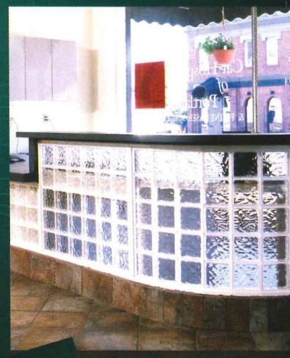
Aluminum mulls were used to connect these flat panels and radius walls together. A flat cap and mounting channel were used to mount the units to the base and the walls. Flat caps were also used to connect the desktop to the top of the panels.
