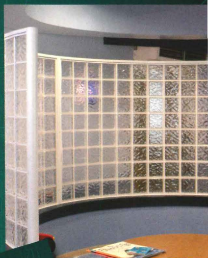
Round caps finished off the ends of this radius wall perfectly. Aluminum mulls were used to connect the three radius walls together, while a flat cap mounted the units to the top of the curved wall.
