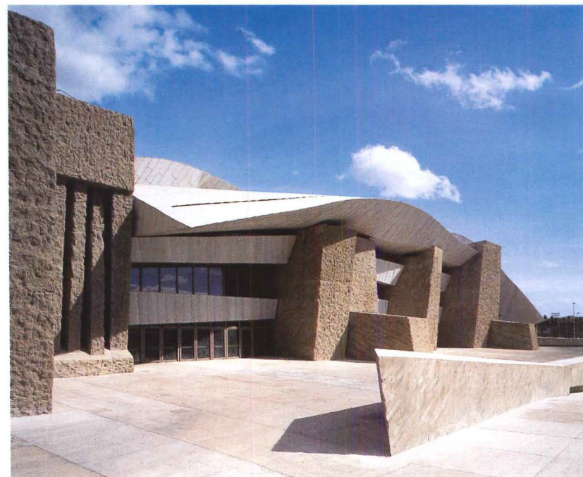
The massive sculptural forms of concrete are mixed with chasnera , a compressed volcanic ash. The complex contrasts dramatically with the town of Adeje, as seen when the center is approached from the southeast (top), and from the main entrance forecourt on the southwest (above).
