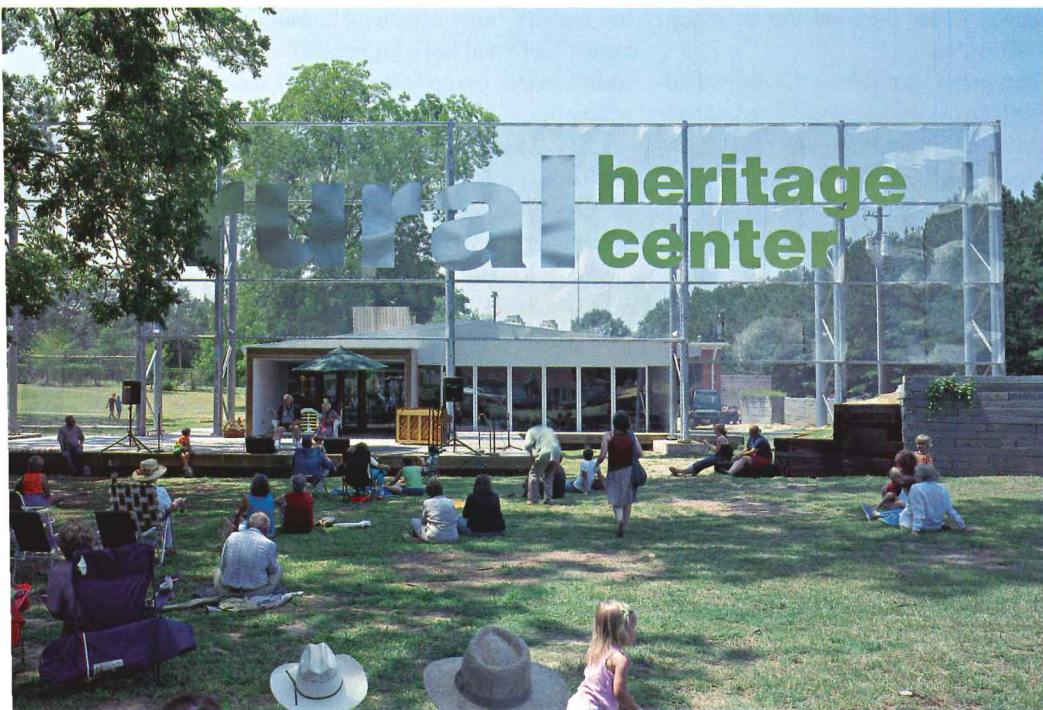
Rural Heritage Center, Thomaston, Alabama: The Rural Studio took an existing 1950s building, renovated it, and expanded it to create this new facility. A 100-foot-high sign made of perforated metal set on vertical trusses gives the building a civic presence and backdrop for an outdoor performance space.
