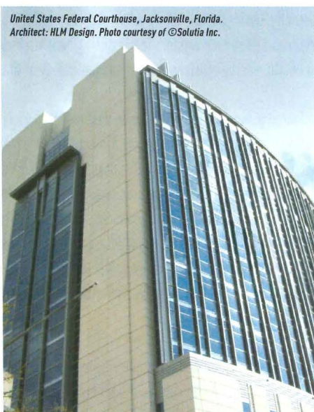
Typical Glazing Retentivity Under Blast Load This courthouse uses insulating laminated units with low-e coatings to address safety and security, and optimize energy performance.
