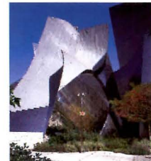
Temporary shield from the glare in L.A.
