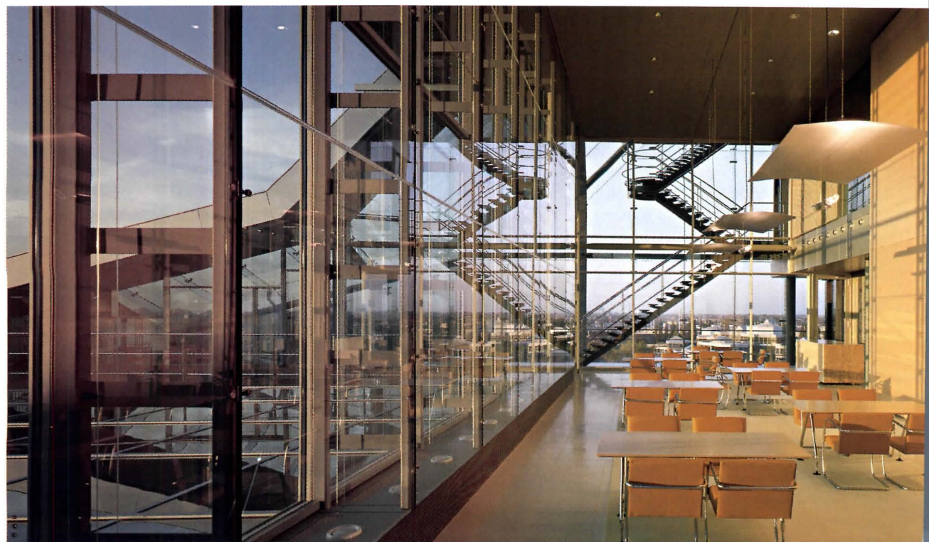
The sloping roof of the restaurant on the seventh floor (opposite, top) is double glass outside and single glass inside, with sunshades in between. The steel load-bearing construction can be seen from one of the two atria (opposite, bottom). Glass stairs connect the ninth and 10th floors (above), used exclusively by the board of directors. Maplewood walls and Mies van der Rohe chairs are featured in the board's stylish dining room on the ninth floor (right).
