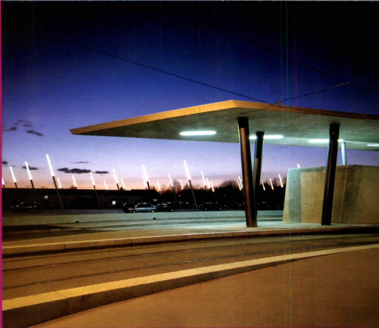
The car park and tram terminal Hoenheim-Nord, in Strasbourg, France, is a kinetic composition of angular light posts, columns, and a folded concrete canopy.
