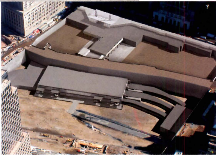
The photomontage (above) depicts the temporary PATH station that will be complete in a year, including an entrance canopy (top) on Church Street.
