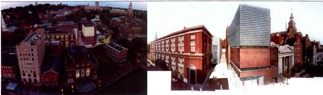
The RISD Center will have studios on the top three glass-enclosed floors.
