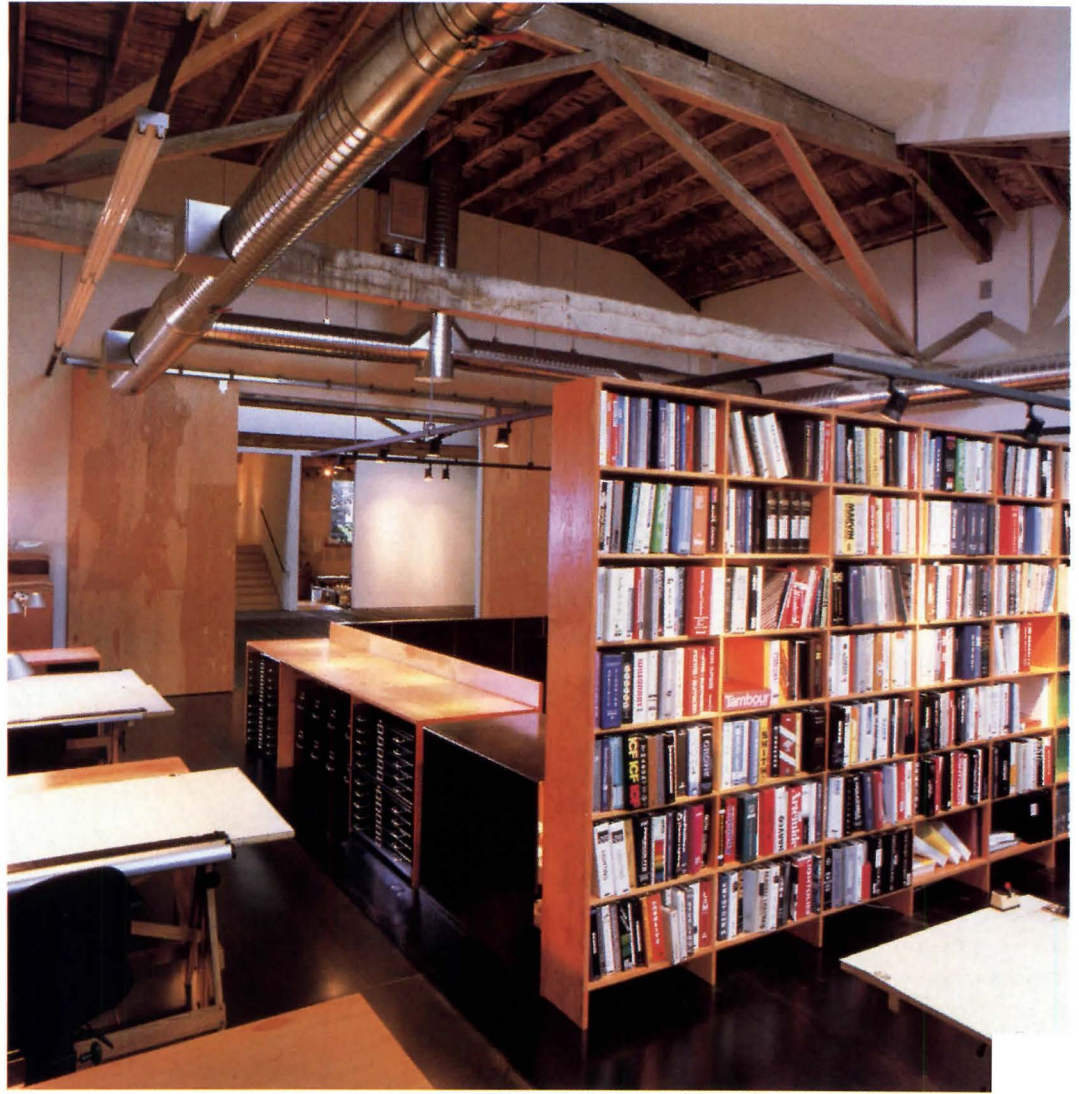
The gallery retains the worn wood-plank floor, with its exposed old-growth wood trusses and decking overhead intact (opposite). A view from the office space at the back of the building looking toward the front (above). Narrow skylights parallel to the front wall cut into the roof to bring light deep inside (below).
