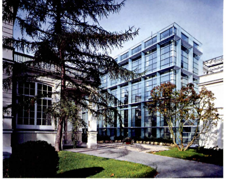
The facade is made of thermally reflective double-glazed units.
