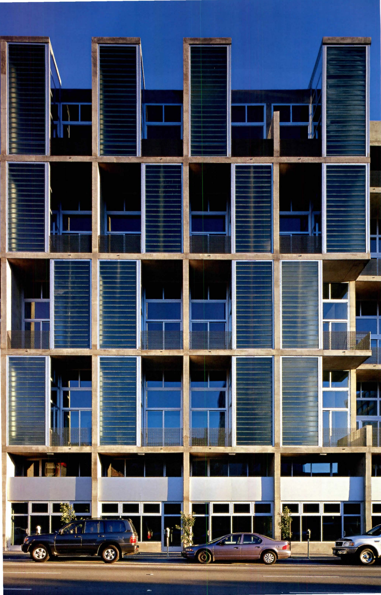
The 200-unit building occupies an entire block south of Market Street (opposite). Each two-story loft facing Folsom Street (left) has an open terrace and a space enclosed on one side by floor-to-ceiling channel glass.
