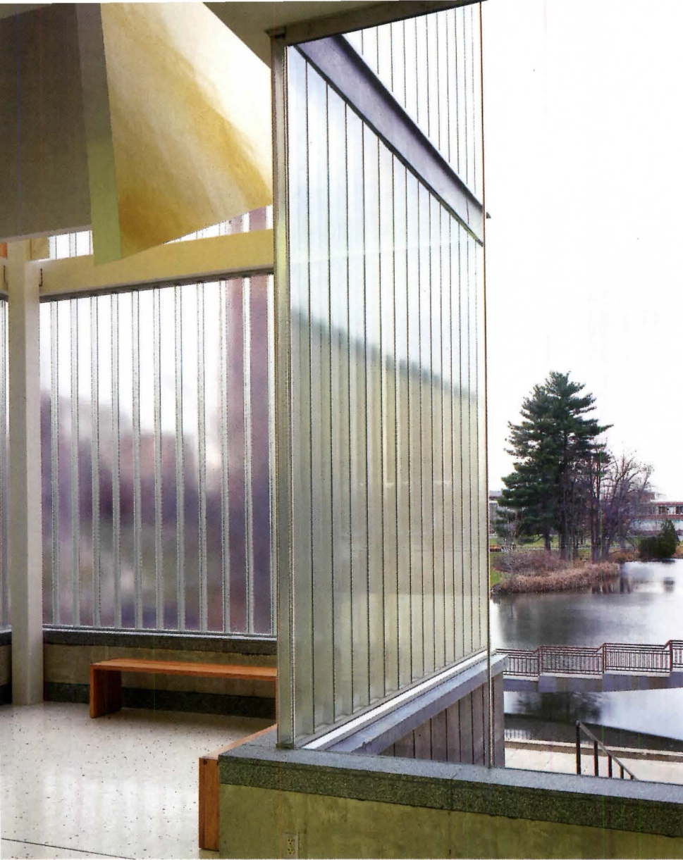
Two types of glass offer differing levels of transparency to direct the viewer's gaze through the building (above and below). Colored lights animate the south elevation at night (below right).
