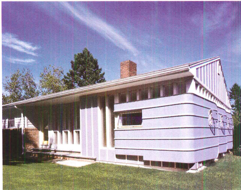
Ranch House Addition, Amagansett, NY, 2001
