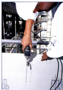
Gypsum/cellulose panels do not cause skin irritation or itch during cutting and handling.
