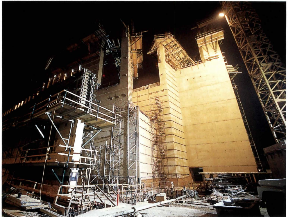
The concrete walls of the Cathedral of Our Lady of the Angels range from one to five feet thick.
