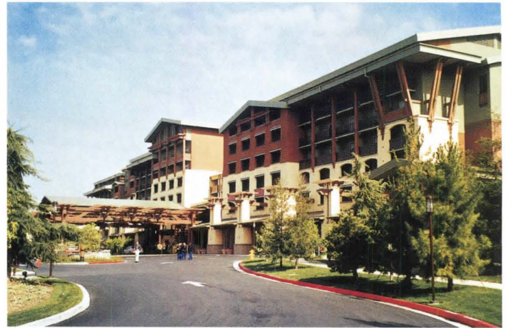
Urban Design Group's Grand Californian Hotel is based on Arts & Crafts design.
