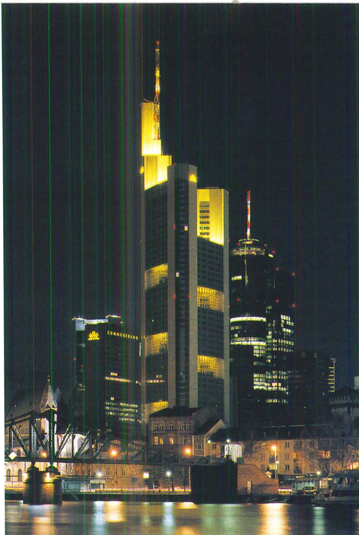
Metal-halide luminaires delineate the interior gardens and perimeter structural columns (details, below) of Frankfurt's Commerzbank Tower (above).
