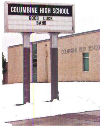
Built in 1973, Columbine High School was typical of its era: sprawling and anonymous.
