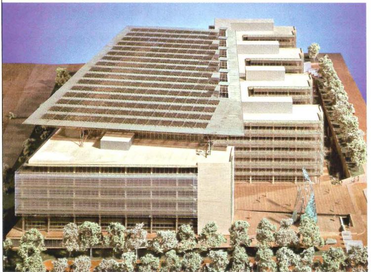
Endesa, implementing passive ventilation, is designed without air-conditioning.
