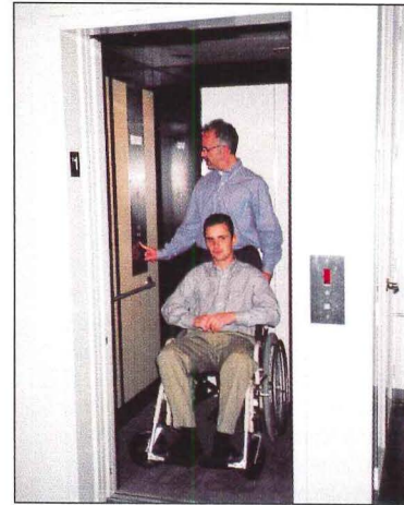
Concord Elevator Inc.
