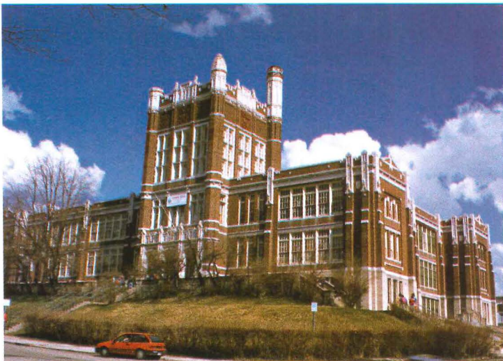
Cincinnati's Hoffman Public School will receive deferred maintenance funds.
