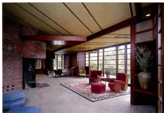
Massive unreinforced chimneys, long window walls, and an open plan (above and left) made the repair and seismic upgrade of the Hanna House difficult.
