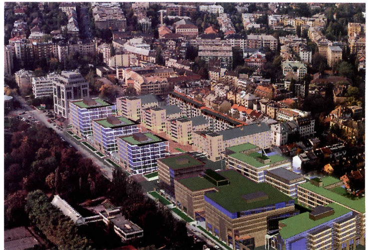
MOM Park, a multiuse complex, is taking shape on a 10-acre site.
