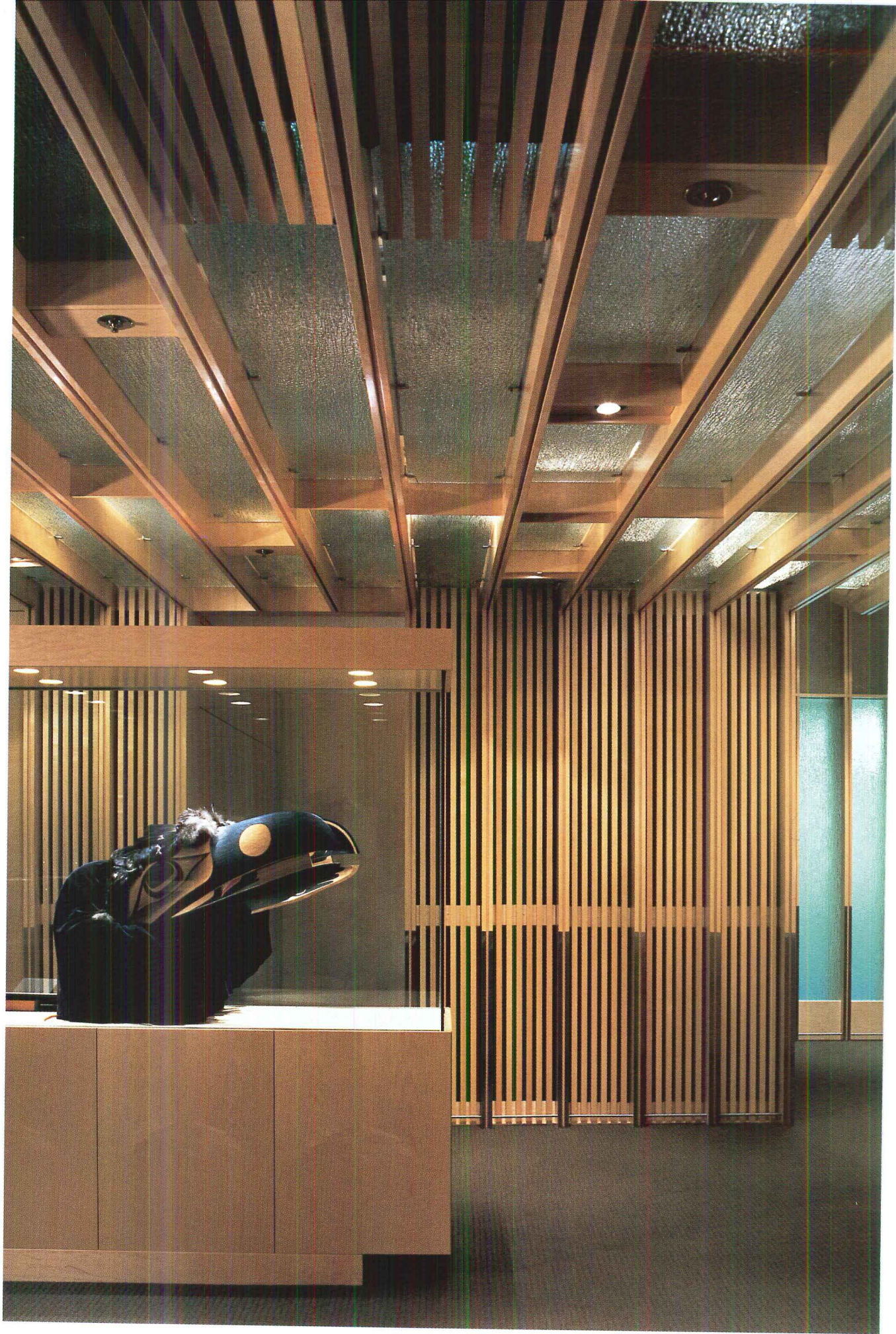
The indirect incandescent lighting, calibrated to evoke daylight, glows through laminated, patterned glass, animating the architects' system of maple ribs and battens (over air outlets and sound-absorption material, as needed). A preset dimming system constantly varies the lighting as if clouds were passing overhead.
