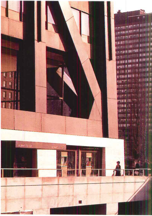
The megascale exposed steel structure with diagonal reinforcing members has a powerful presence on the exterior (above and right), and at key points on the interior (below).
