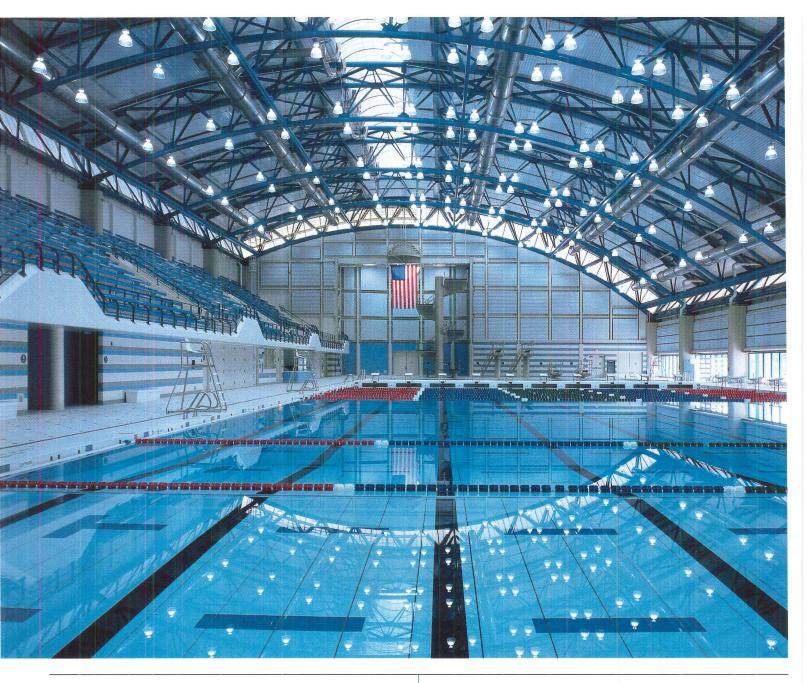
is no permanent seating, walls made of glass doors can slide to one side. Metal wall panels above the doors can then be pivoted upward until they are horizontal, creating an opening 30 feet wide by 19 feet high where bleachers can be installed. Permanent stretched-fabric sunshades protect spectators.
