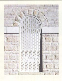
A stone panel, carved by sculptor Alan Tollackson, was based on Kent Bloomer's maquette of prairie plants. As the shadow line (photo left) and section (far left) indicate, the panel's lower two-thirds are set into a battered veneer wall. What appear to be blocked-up arched openings never actually contained windows: they were constructed on the building's exterior to maintain the rhythm of a series of real openings when structural loading of a wall prevented cutting a window.
