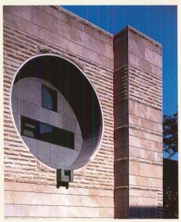
A cylindrical surround of greenstone highlights windows in the school building's vestibule. To create the cylinder's wall, the architect pinned segments of honed stone to an octagonally shaped backing of poured concrete with stainless-steel hardware.
