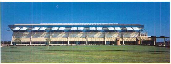
The pool level is on grade with the building's south elevation (above and left). To open up this level for extra seating, the glass doors next to the patio can slide to one side and the metal paneled wall above can pivot up and away from the building until it is horizontal. The north side of the building (below left) is at the same level as the spectator seating. Stretched fabric sunshades protect both sides of the building from direct sunlight during the summer.
