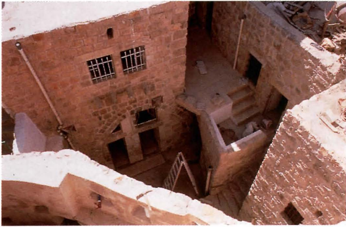
Rehabilitation of Hebron Old Town, Hebron, Israel Planners/Conservators: Engineering Office of the Hebron Rehabilitation Committee
