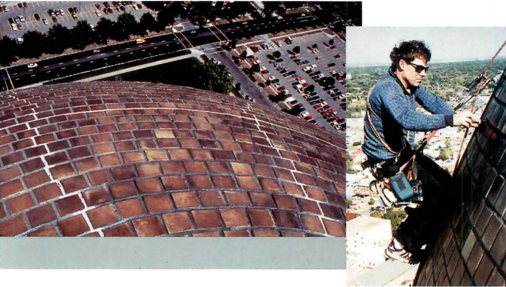
RAPPELLING FROM THE SOWER, A STATUE atop the capitol dome (left), field inspectors performed visual inspections and applied nondestructive testing methods to examine cracks in the dome (far left) and assess the tower's condition.
