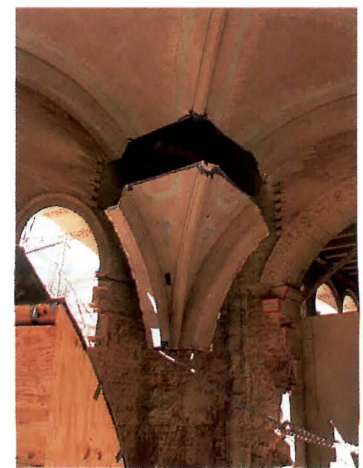
Removing the corners of the vaulted ceilings beneath the towers provided access to supporting piers.
