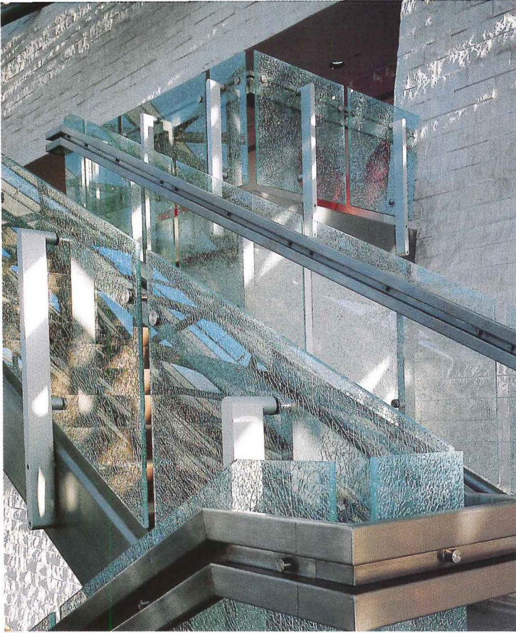
Glass panels, which have a layer of fractured glass sandwiched between two unbroken layers, reinforce the shimmering effect of daylight streaming through the crystalline structure of the lobby (left and above).
