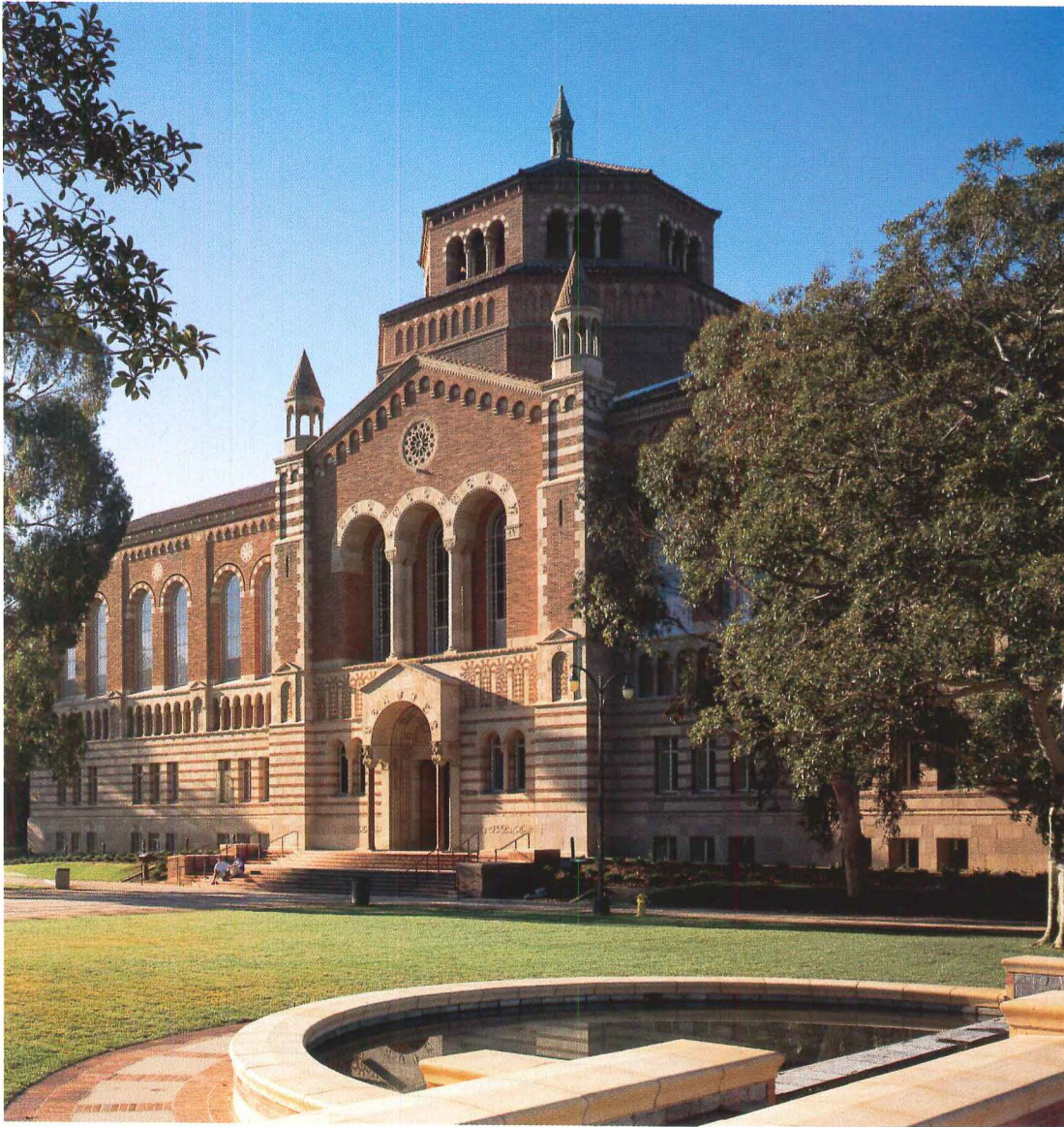
Powell Library Renovation University of California, Los Angeles Owner: University of California Architect: Moore Ruble Yudell Architects & Planners
