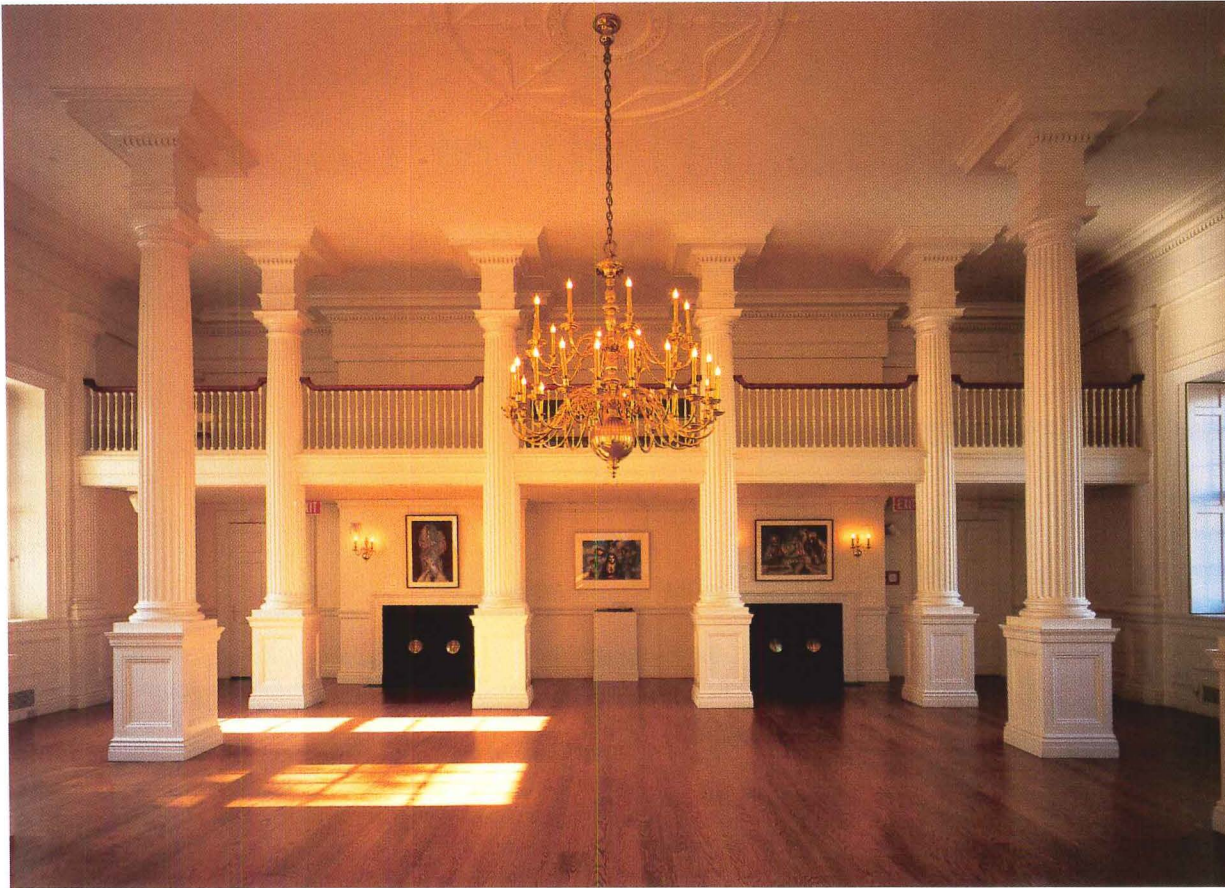
In 1920 the State Supreme Court room was turned into a conjectural Bulfinch interior with bold Doric columns. Its subtle, white-on-white paint treatment, spoiled by uniform white painting in the 1970s, was restored. Since it was impossible to re-create an earlier form of this room—or the first- and second-floor lobbies—it was returned to its 1920 state, serving as an example of 20th-century revivalism.
