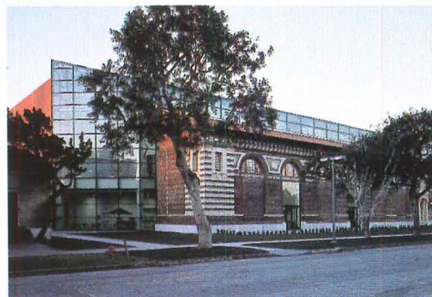
The center of the historic Ahmanson facade was rebuilt with salvaged brick (top) and integrated with the new building (above), which restored the north perimeter of the seven-acre 1928 Rose Garden (right).
