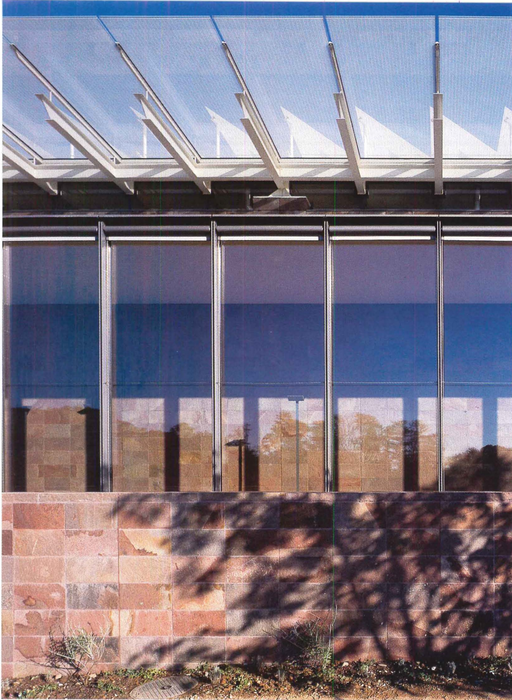
Above: The top of the curtain wall at the winter garden is held well beneath the cantilevered glass roof panels. Left: Layered stone walls enclosing service spaces buffer the museum from the street. Top right: The bulk of the building appears to emerge from the agricultural landscape. Bottom right: Layered walls anchor the west elevation.
