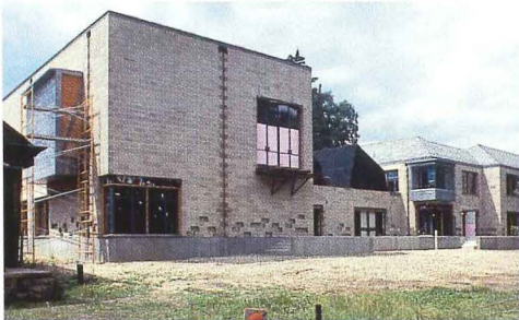
Addition to Brookside Lower School
