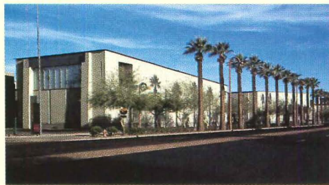
Phoenix Art Museum, nearing completion, by Tod Williams and Billie Tsien.
