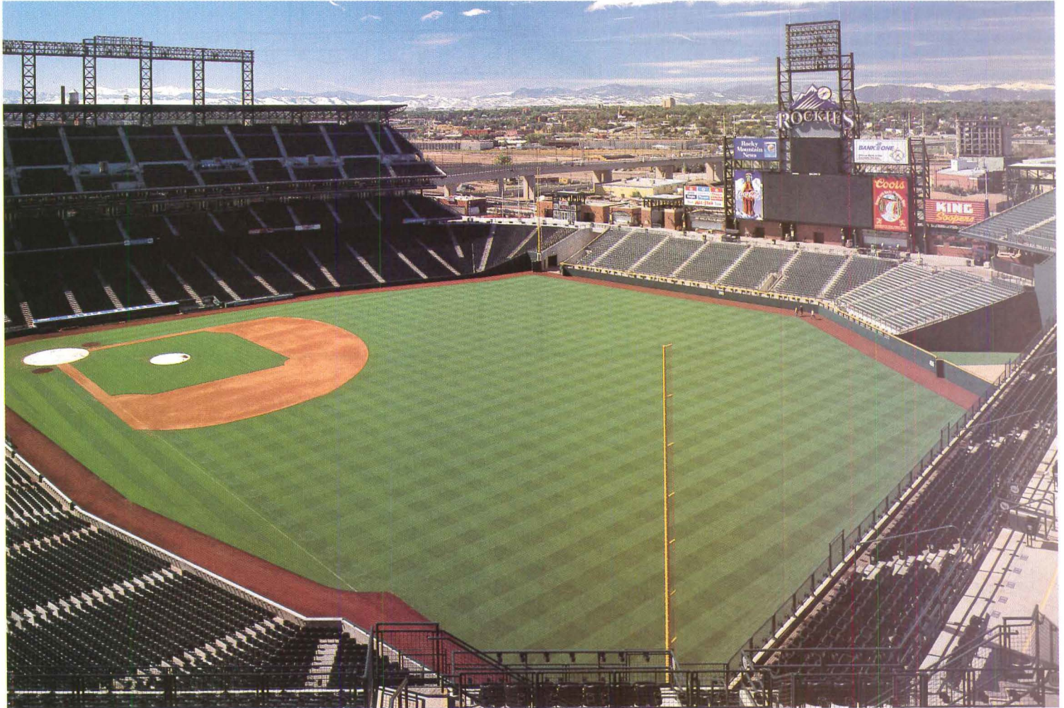
The main and side entrances to Coors Field show (opposite top photos) how HOK Sport has integrated materials and traditional patterns to create the feel of an old-time ballpark. Inside, the facility has all of the modern amenities (above). Sited on the old Union Pacific yards, (opposite) the ball park is woven into existing traffic patterns, and has brought new life into Denver’s lower downtown.
