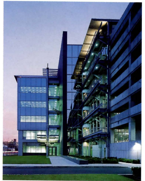
An attached poured-concrete parking garage (above, foreground), is set back from the office building's street facade to reveal the blue-brick wall that separates open, flexible "backhouse" operations space from fixed administrative "fronthouse" functions facing the public, and including the main entrance (top).
