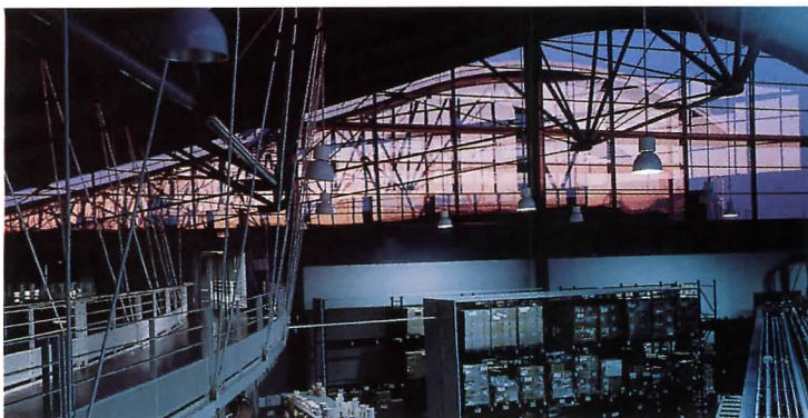
The architects and engineers used structures and materials to make the factory's interior as light and open as possible. For example, the curtain wall at the building's gable ends works with the bulging form of the roof to bring sunlight into the production area (left and above left). A second-story walkway is suspended from the roof and overlooks the manufacturing floor (above right).
