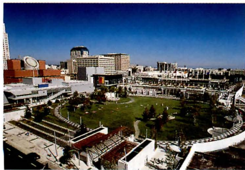
In front of the Botta-designed museum is MGA Partners' $23-million Yerba Buena Esplanade, which links Center for the Arts buildings by James Stewart Polshak (right in photo) and Fumihiko Maki (left).
