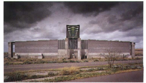
A 480-foot-span steel truss dominates the east facade (above). The roof is hung from the truss, creating a flexible two-acre interior space. All columns line the exterior except for two interior supports, which separate garbage transfer and recycling areas. An outdoor amphitheater between offices is used for public educational events (opposite).
