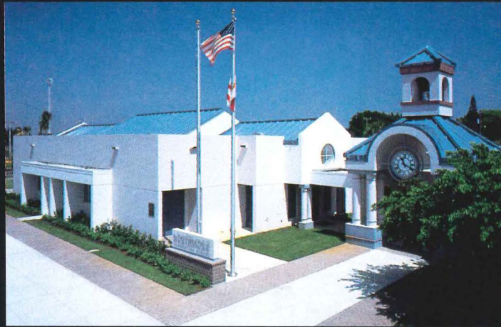
Northmore Elementary School Lantana, Florida
