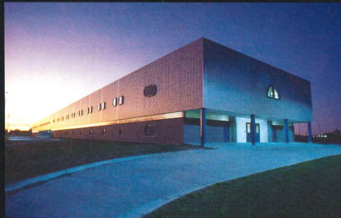
Turner Elementary/Middle School Shreveport, Louisiana
