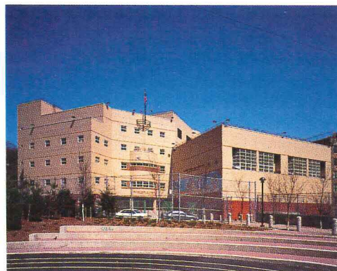
The west facade (opposite) curves away from Broadway to keep classrooms from the noise of the street. The school looks onto Fort Tryon Park in northern Manhattan (top). Most students enter the school from the south, where a playground sits across the street (above).
