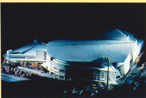
The Kiel Arena's generous overhangs cantilever from the main trusses.
